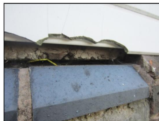
Photo 6: Gaps beneath damaged fascia
