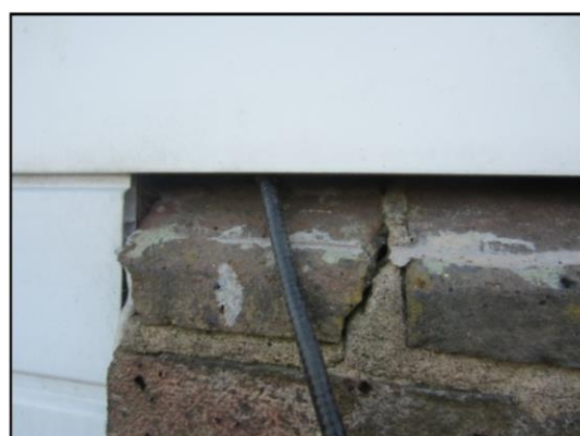
Photo 7: Inspection of gaps behind fascia with borescope.
