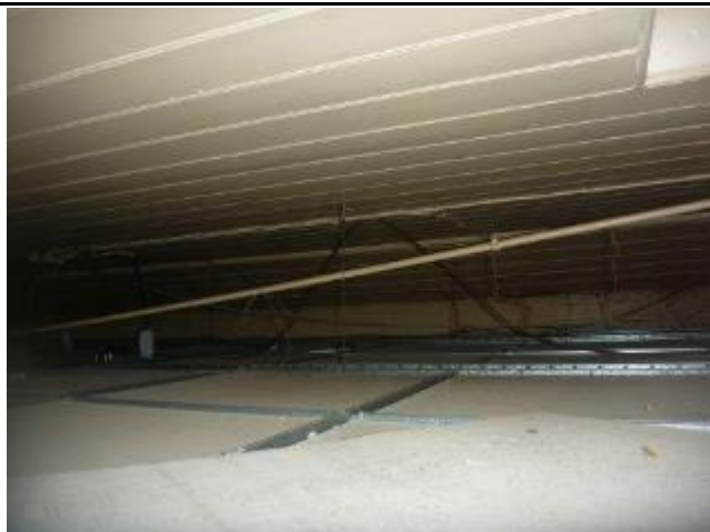
Photograph 9.25: Building 1, section 1c showing vaulted ceiling above suspended ceiling.
