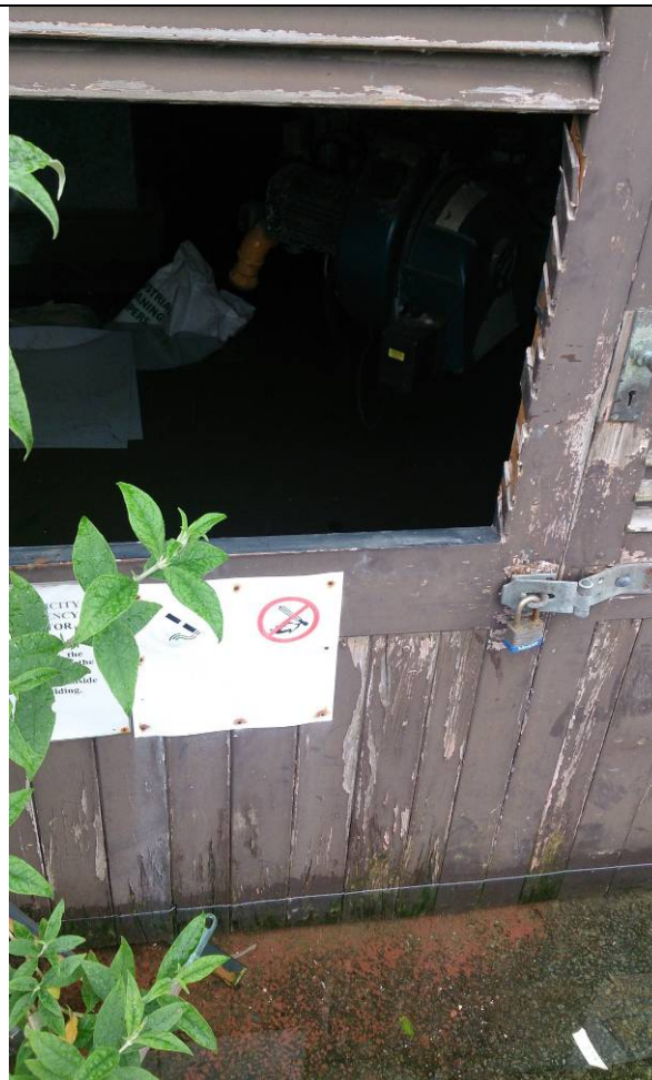
Entrance to boiler house, flooded and warning of asbestos
