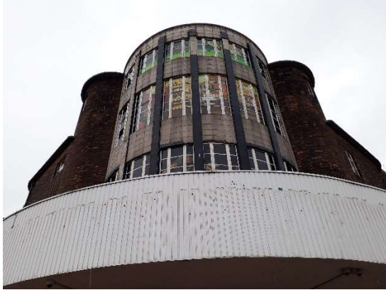
Close view of the building's rotunda and the poor condition of the cement-based tiles.
