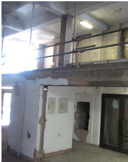
Photo 5 – existing column to side of entrance that would become freestanding and clad in salvaged stonework
