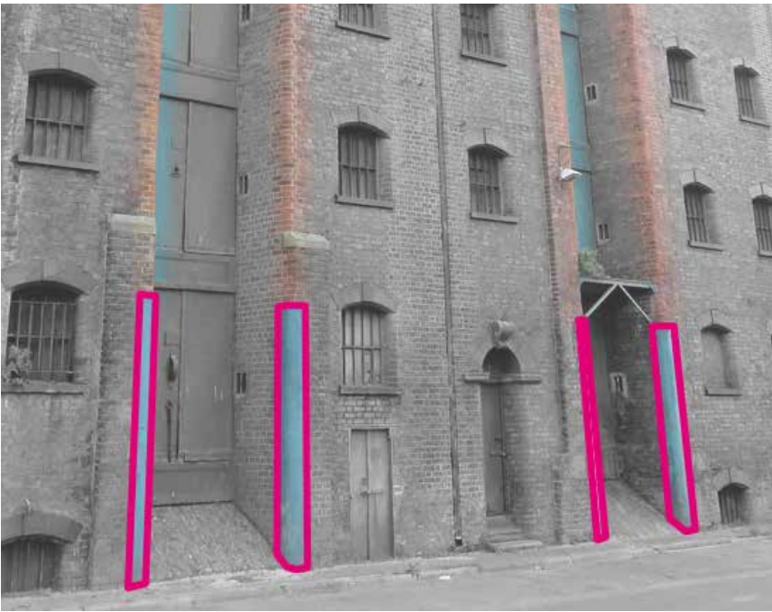
Cast iron bumper guards will be used at the base of the concrete/brick columns to emphasize buildings' access.
