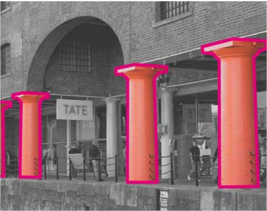
Round pigmented concrete columns as a reference to Albert Dock's cast iron columns and lifting bay rounded corners.
