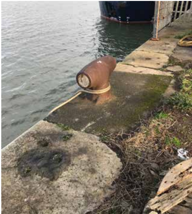
Figure 3.5.6: Mooring bollard
