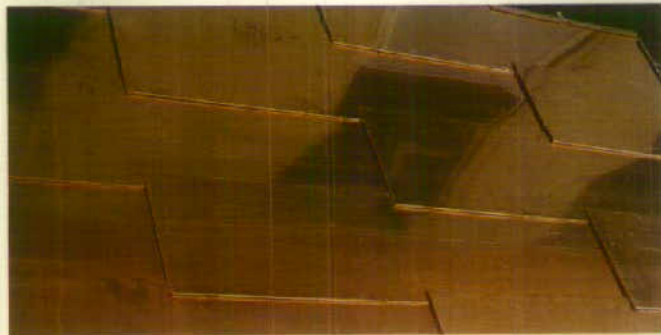
New copper shingles
