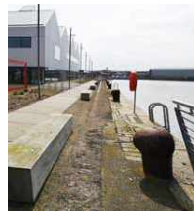
Mooring bollards in-situ at Wirral College
