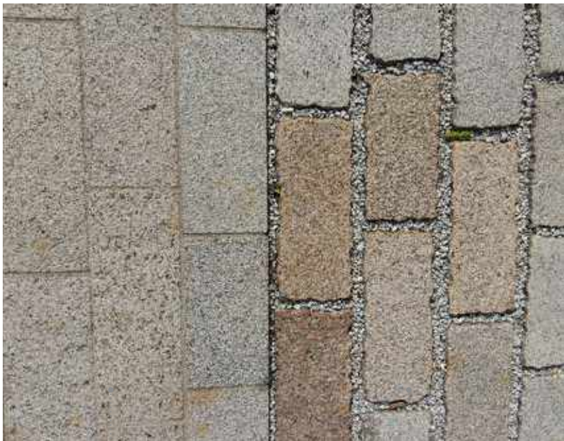
New granite flags with sawn edges and narrow joints
