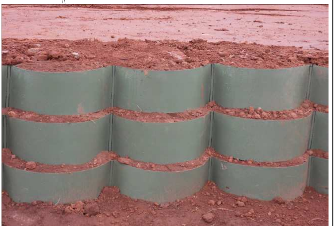
Panels are stepped back from the front face of the panels below by a specified amount depending on the required slope angle. A 100mm finished step-back equates to a 68° slope.
