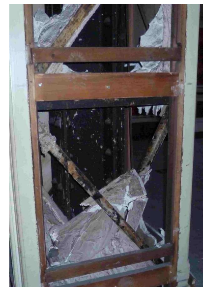
Existing steel structural columns
