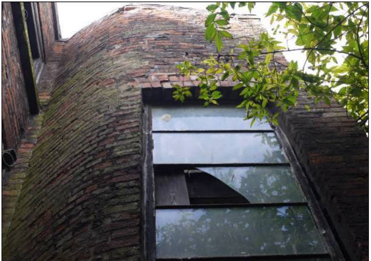
15. Bullnose form of the outrigger of 93
