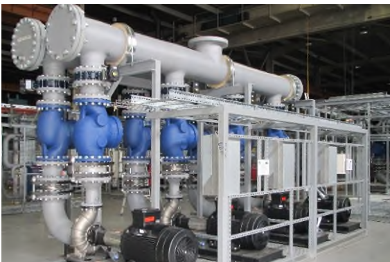
Example modularised MEP plant skids
