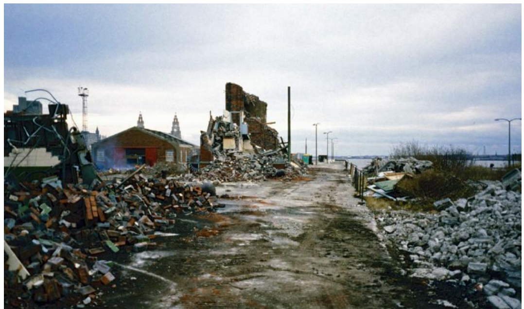
Figure 9.14: 1999 showing the demolition of the accumulator building used in conjunction with the river lock at West Waterloo Dock. The infilled lock is to the right of the image (John Luxton).
