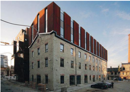
2 storey roof extension on brick building
