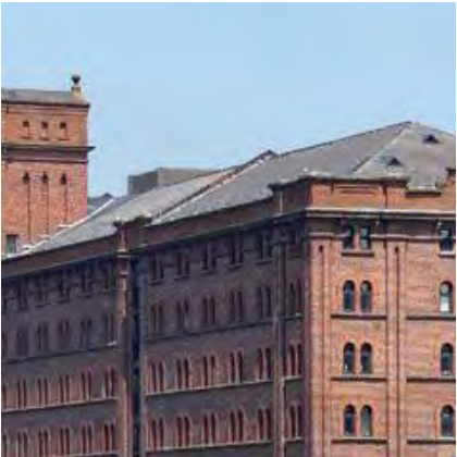
Change in material above brick parapet on Albert Dock Warehouse and Waterloo Warehouse
