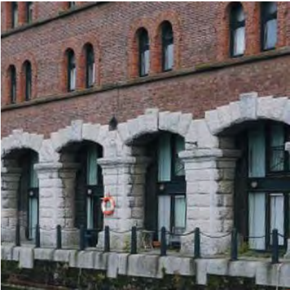
Segmented arches on the Merseyside Maritime Museum and Waterloo Warehouse
