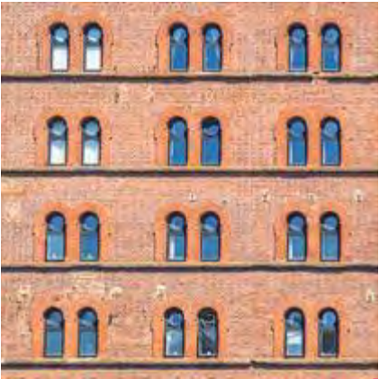
Horizontal brick banding on Stanley Dock Tobacco Warehouse and Waterloo Warehouse
