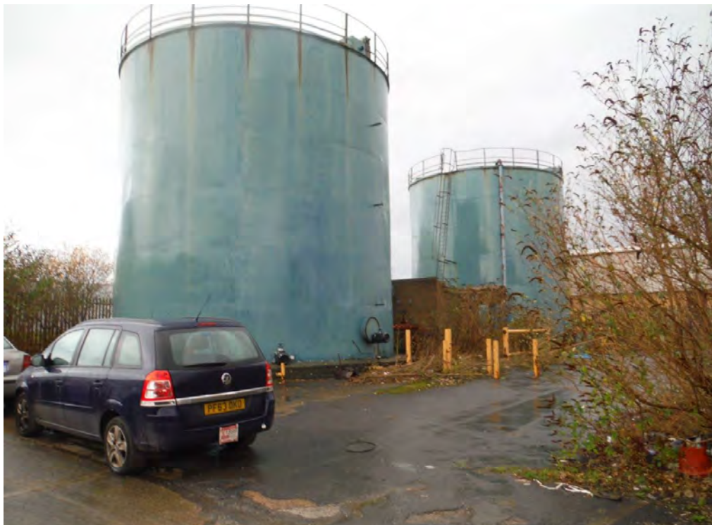
Figure 18: Large tanks to the north of the site.
