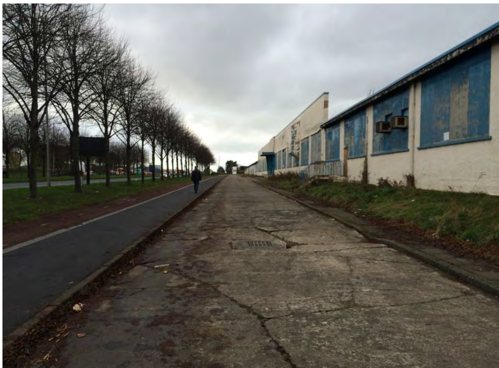
Figure 10: Road along southern boundary.
