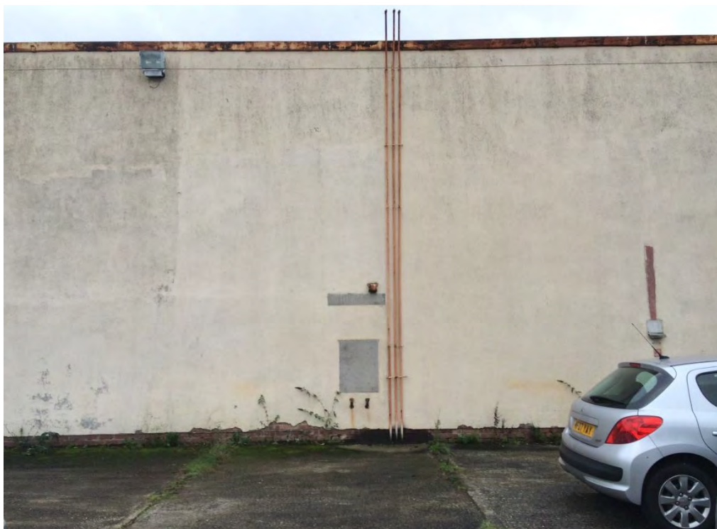
Figure 2: 3 x breaker pipes potentially from underground tanks in west of site.
