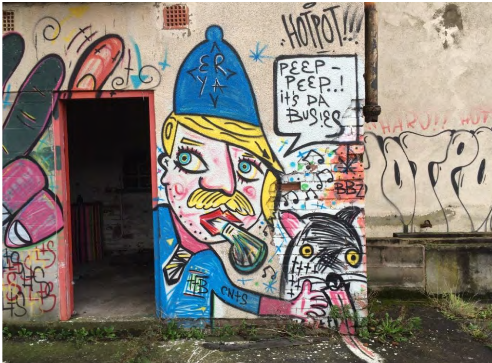
Figure 9: Chemical store room in west of site.
