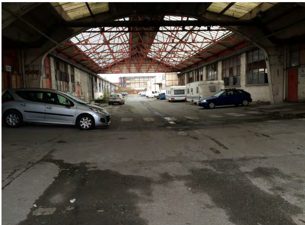
Figure 4: Inside building looking west.
