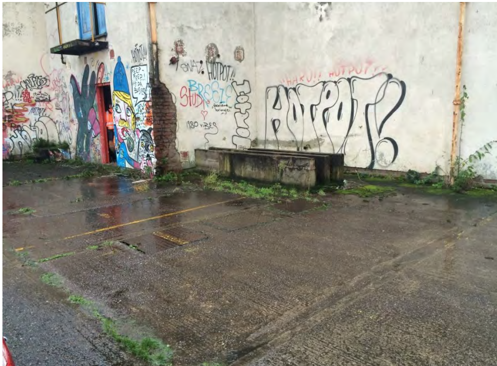
Figure 1: Interceptor drain and possible tank stand in west of site.
