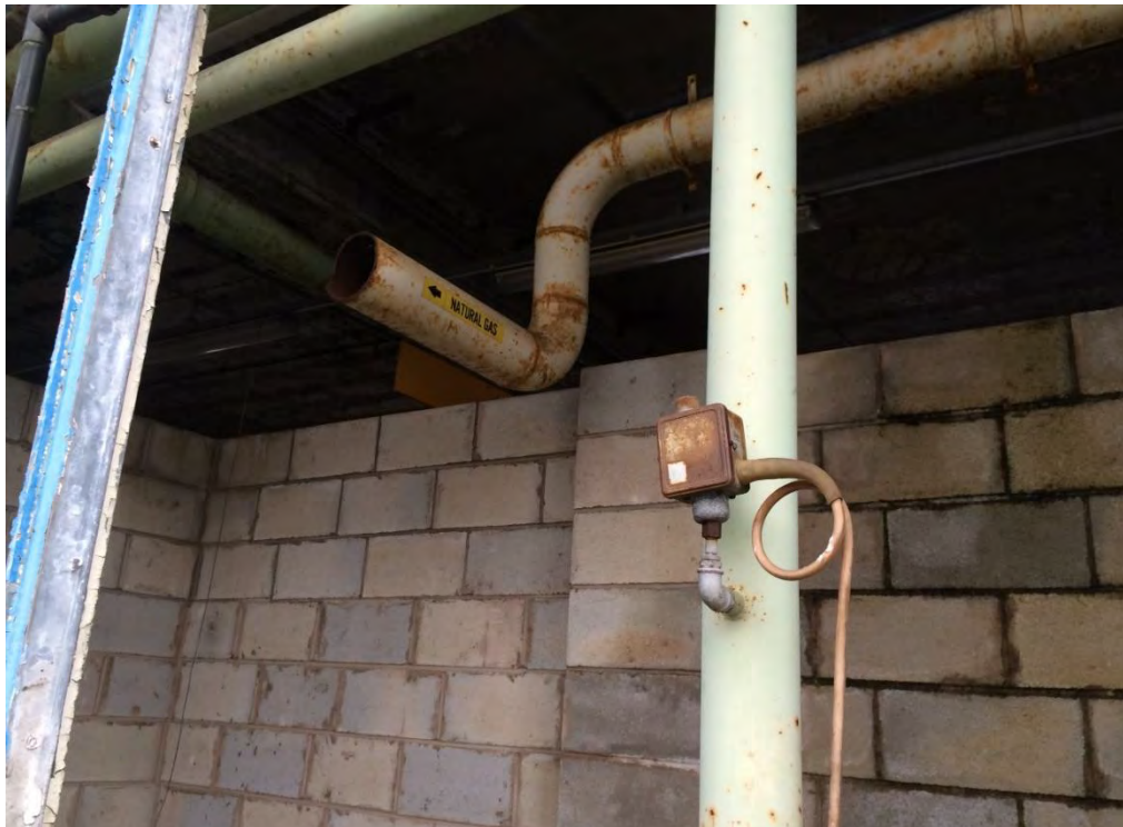
Figure 7: Plant room noted in eastern section of northern building.
