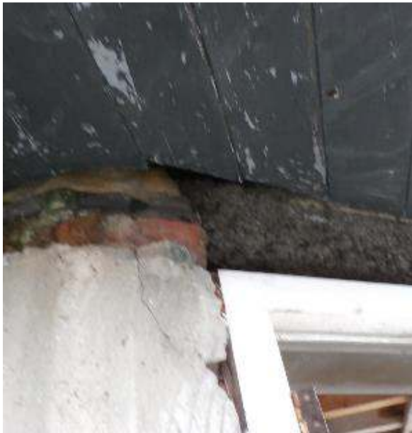
Figure 20 Gaps beneath the timber panels on the dormer style roof adjacent to the bay window and at the building eaves providing potential access / egress to further suitable cavities.
