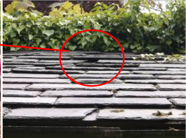
Gaps at lifted & slipped roof slates
