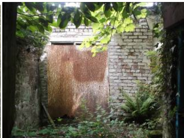
Eastern elevation 8 with slipped metal sheeting
