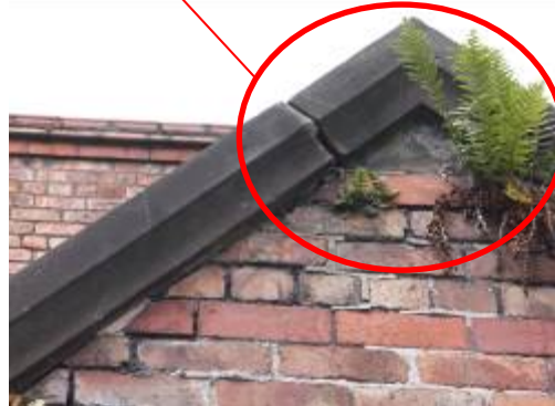
Gaps at the capping stones
