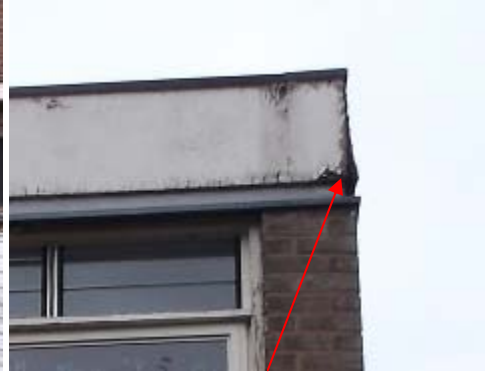
Lifted fascias on eastern elevation
