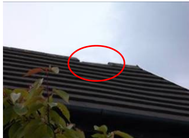
Missing ridge tile on 1b
