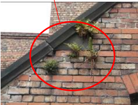
Gaps in the brickwork
