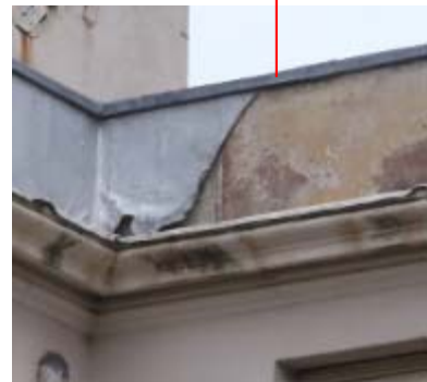
Gaps under lead flashing
