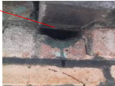
Gaps at the roofline
