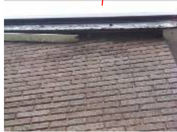
Rotted wooden soffit
