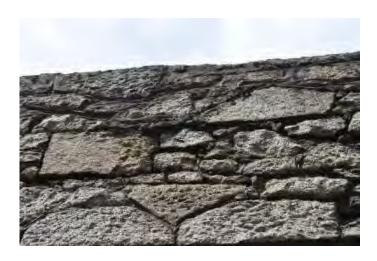
Area of repointed coping. Mortar loss and cracking of stonework below.
