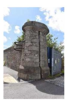
Signage fixed to pier with ferrous staining of the stonework. Plant growth to upper stonework elements. Gate present in recess.
