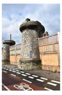
Central Lodge – Formed of random coursed granite stonework of similar construction to the main wall. Dressed plinth and projecting cornice, 2No windows facing the road have been blocked in and evidence of chimney at roof level. The base of the lodge is 4575 x 3080 in plan.
