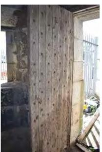
Internal view of the 2No windows facing the road. Blocked in however stonework to opening appears in sound condition.
