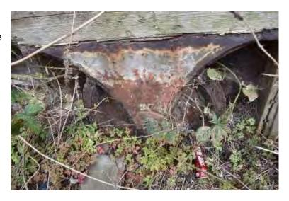
Timberwork is degraded especially at low level however a conservation repair could be undertaken to retain historic elements of the gate in sound condition.
