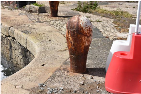
Bollard removed by over-coring removing bollard and surrounding concrete.
