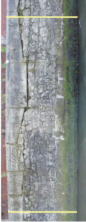
A133 Chainage 640 to 645m
