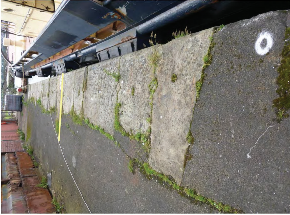
Figure A138a - Bramley Moore: Coping Chainage 665 to 670m
