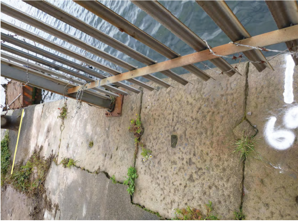
Figure A143a - Bramley Moore: Coping Chainage 690 to 695m
