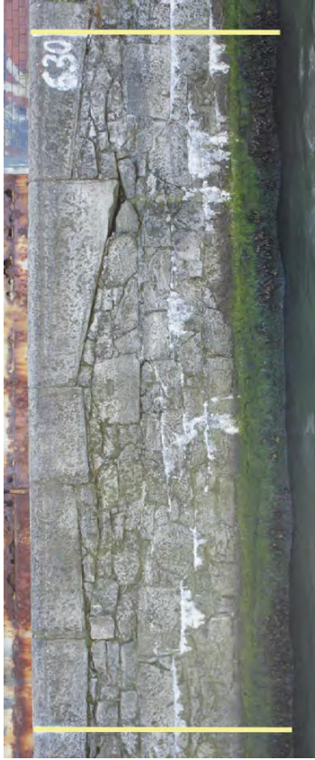
A130 Chainage 625 to 630m
