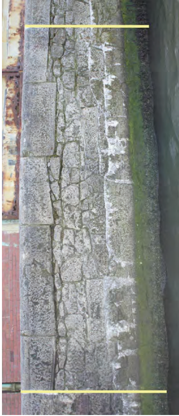
A129 Chainage 620 to 625m
