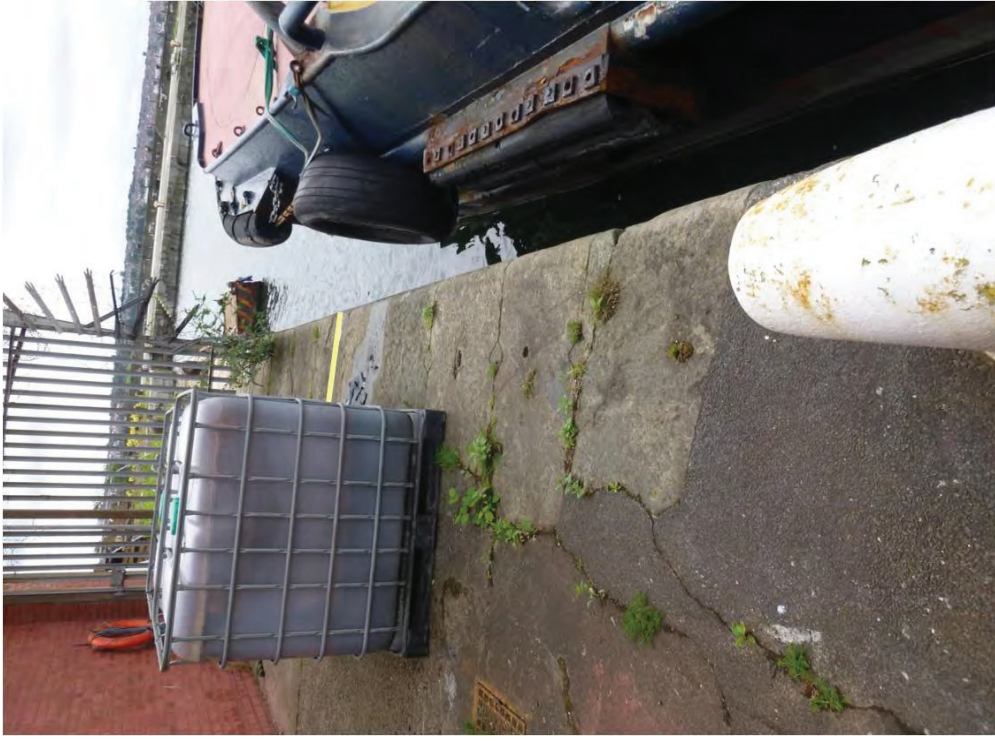
Figure A141a - Bramley Moore: Coping Chainage 680 to 685m
