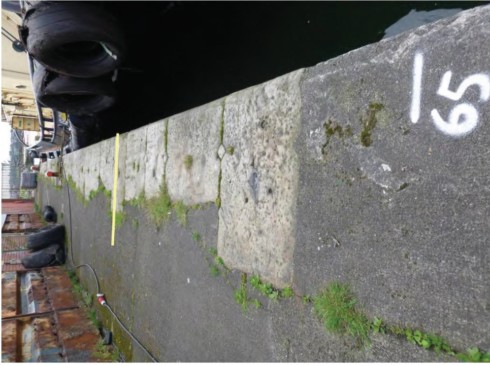
Figure A135a - Bramley Moore: Coping Chainage 650 to 655m
