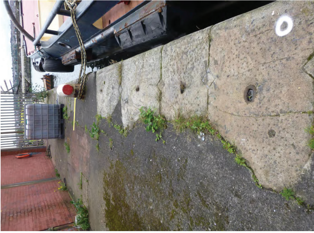
Figure A140a - Bramley Moore: Coping Chainage 675 to 680m
