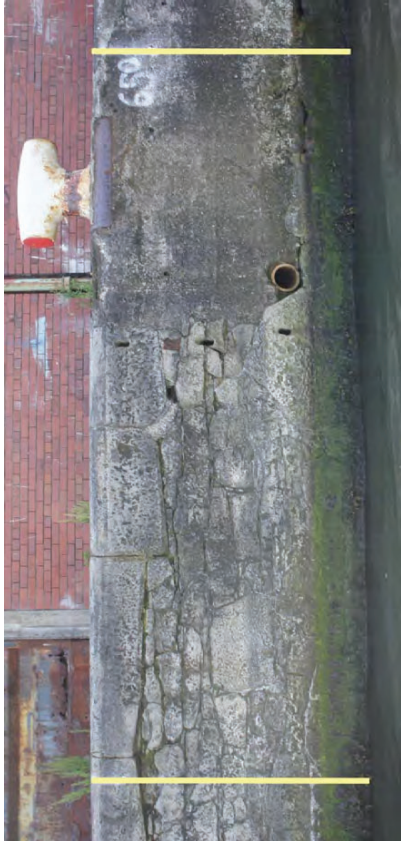
A134 Chainage 645 to 650m
