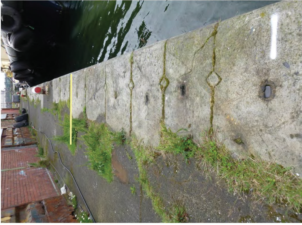
Figure A133a - Bramley Moore: Coping Chainage 640 to 645m
