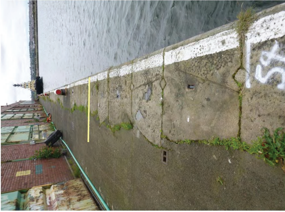
Figure A113a - Bramley Moore: Coping Chainage 540 to 545m
