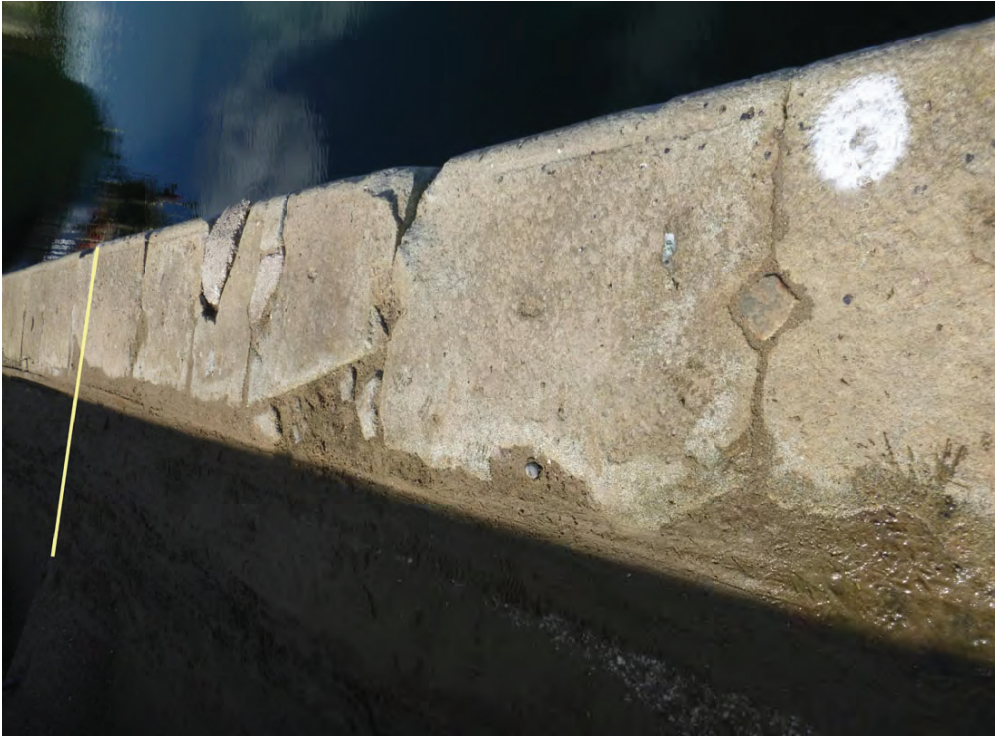
Figure A82a - Bramley Moore: Coping Chainage 385 to 390m
