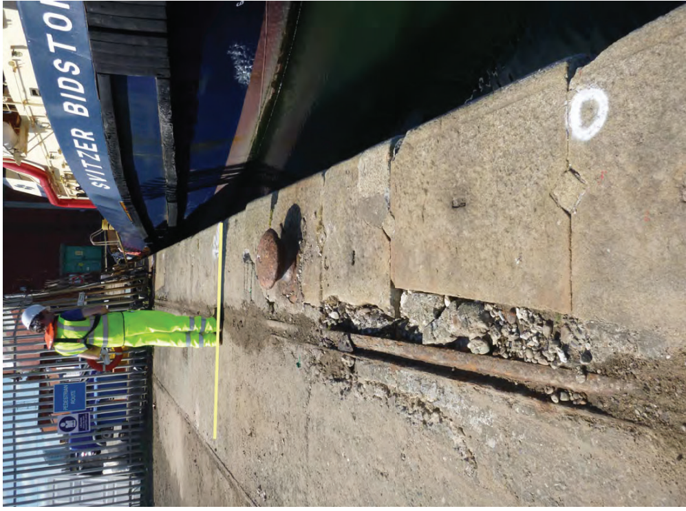
Figure A88a - Bramley Moore: Coping Chainage 415 to 420m
