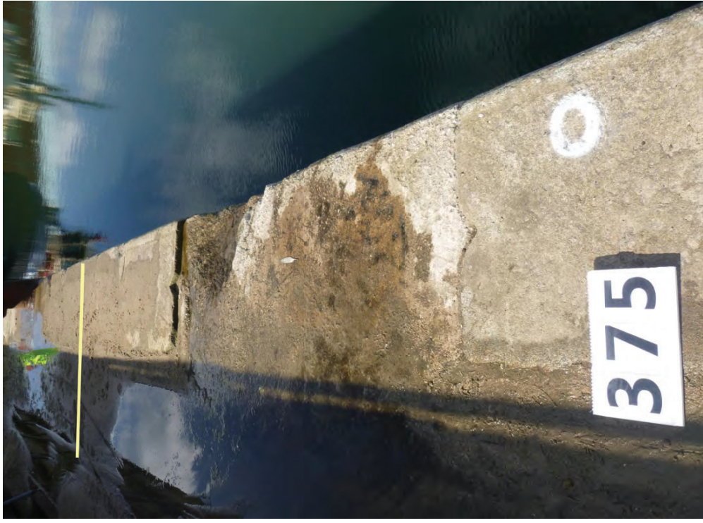
Figure A80a - Bramley Moore: Coping Chainage 375 to 380m
