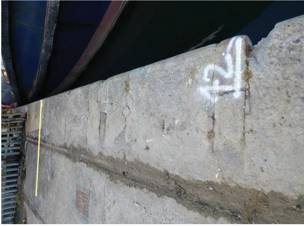
Figure A89a - Bramley Moore: Coping Chainage 420 to 425m
