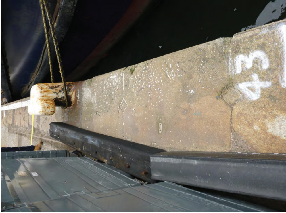
Figure A91a - Bramley Moore: Coping Chainage 430 to 435m
