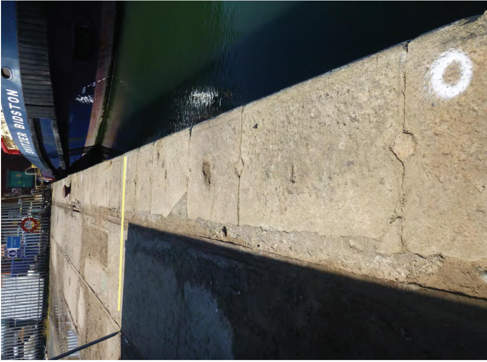
Figure A86a - Bramley Moore: Coping Chainage 405 to 410m
