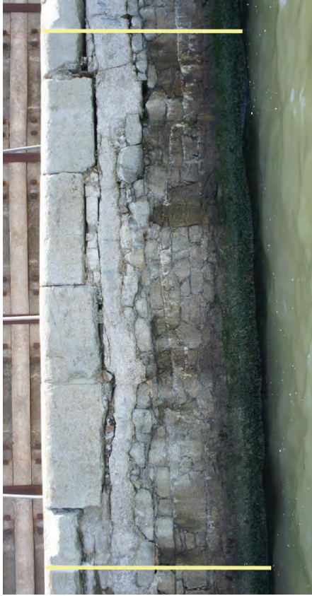
A83 Chainage 390 to 395m
