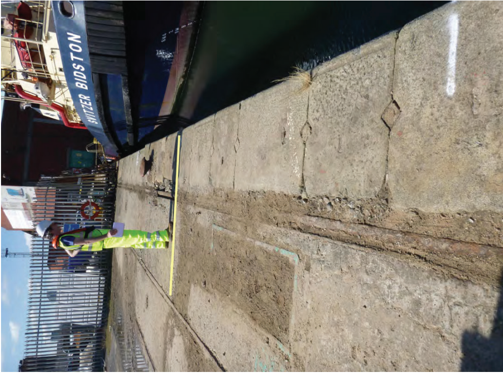
Figure A87a - Bramley Moore: Coping Chainage 410 to 415m
