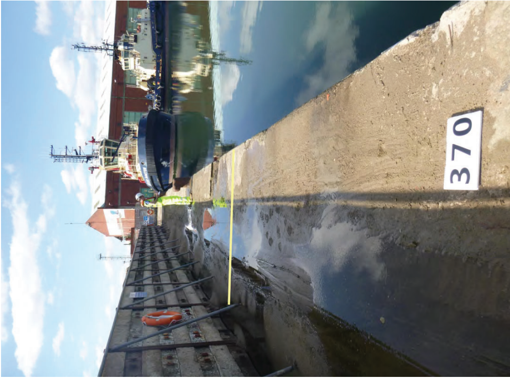
Figure A79a - Bramley Moore: Coping Chainage 370 to 375m
