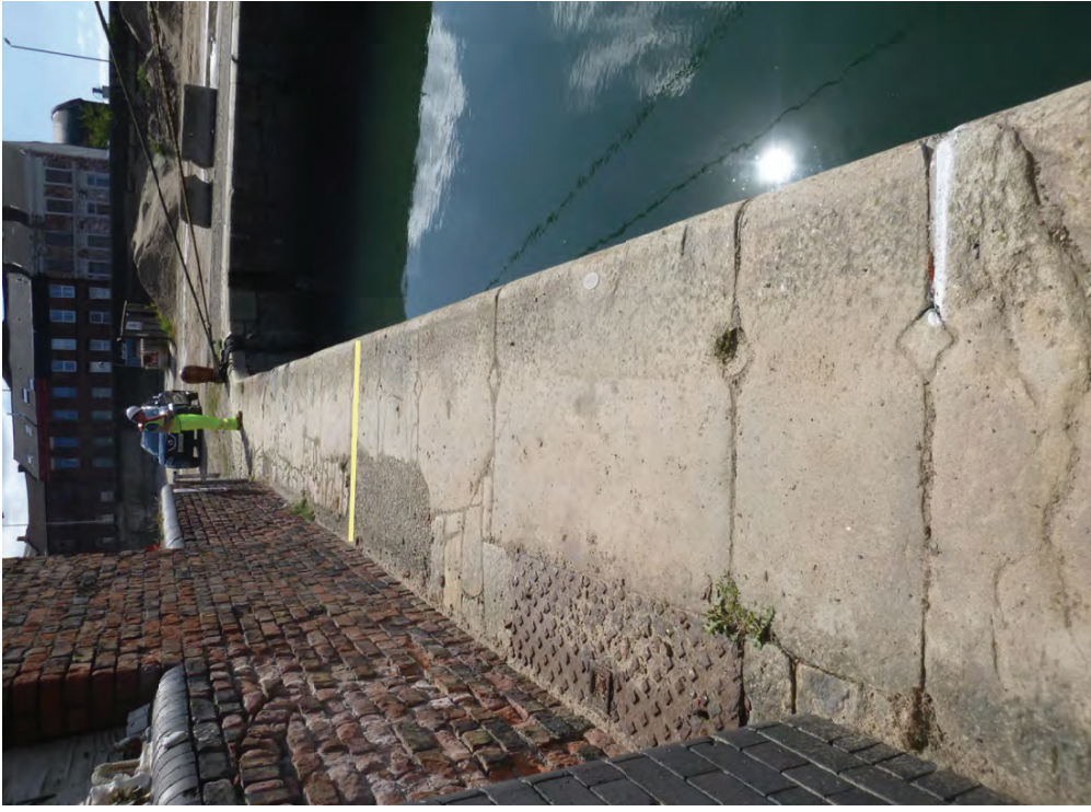
Figure A67a - Bramley Moore: Coping Chainage 310 to 315m
