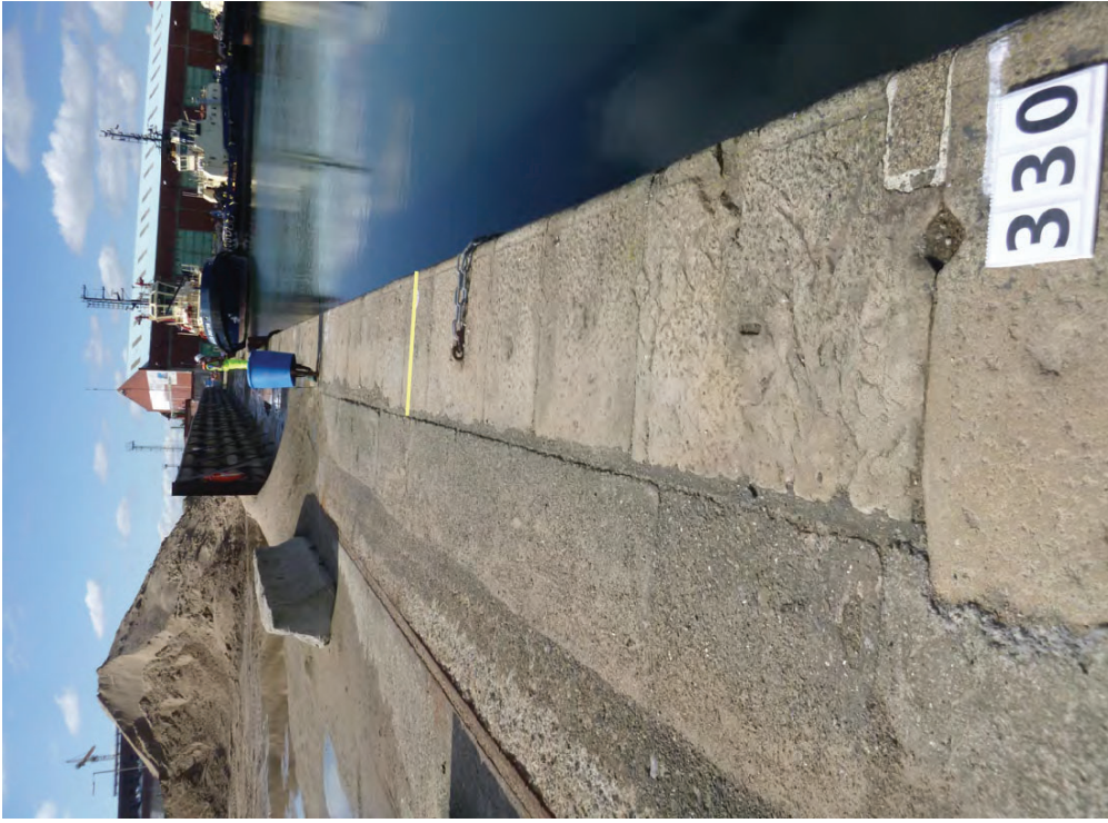
Figure A71a - Bramley Moore: Coping Chainage 330 to 335m
