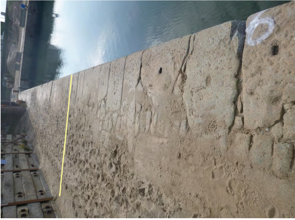
Figure A62a - Bramley Moore: Coping Chainage 285 to 290m
