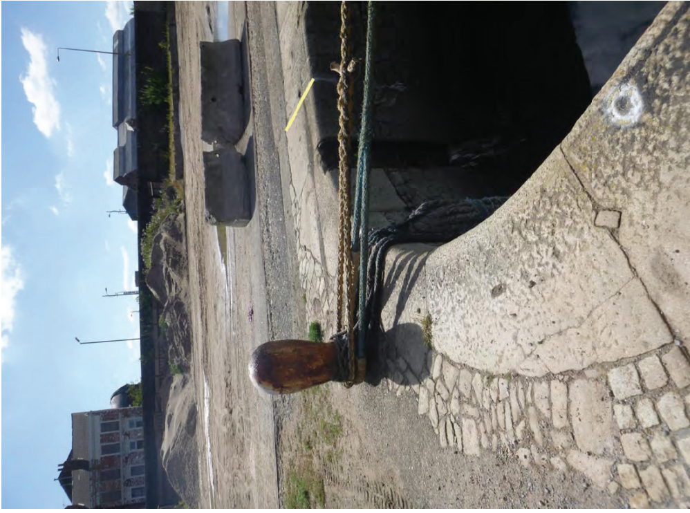
Figure A70a - Bramley Moore: Coping Chainage 325 to 330m
