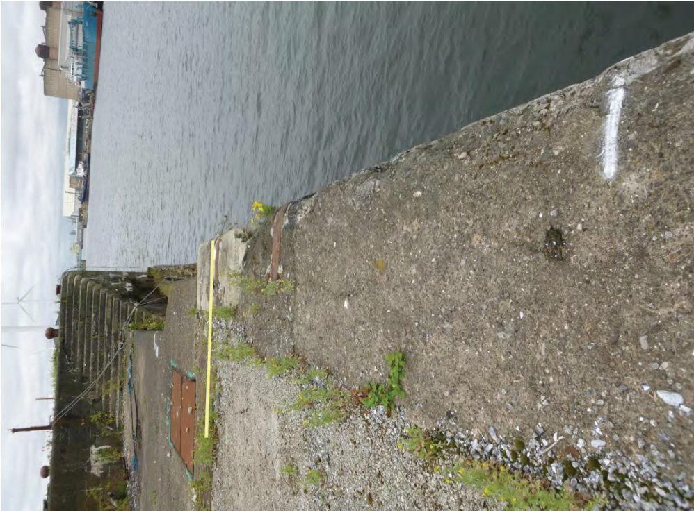
Figure A196a - Bramley Moore: Coping Chainage 955 to 960m
