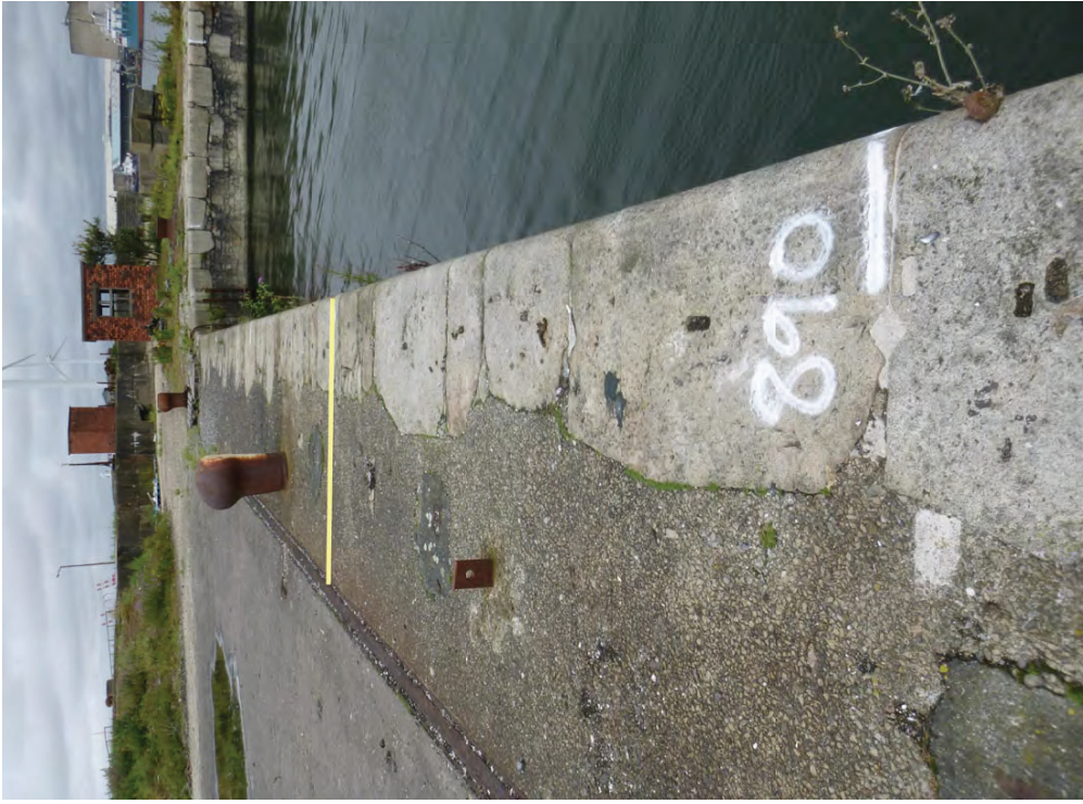
Figure A183a - Bramley Moore: Coping Chainage 890 to 895m
