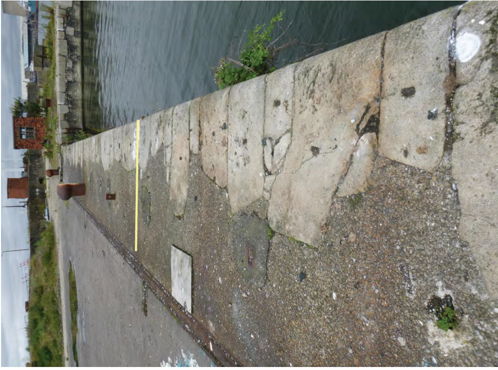
Figure A182a - Bramley Moore: Coping Chainage 885 to 890m
