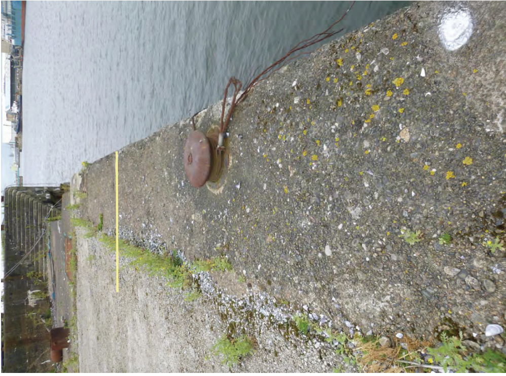
Figure A195a - Bramley Moore: Coping Chainage 950 to 955m
