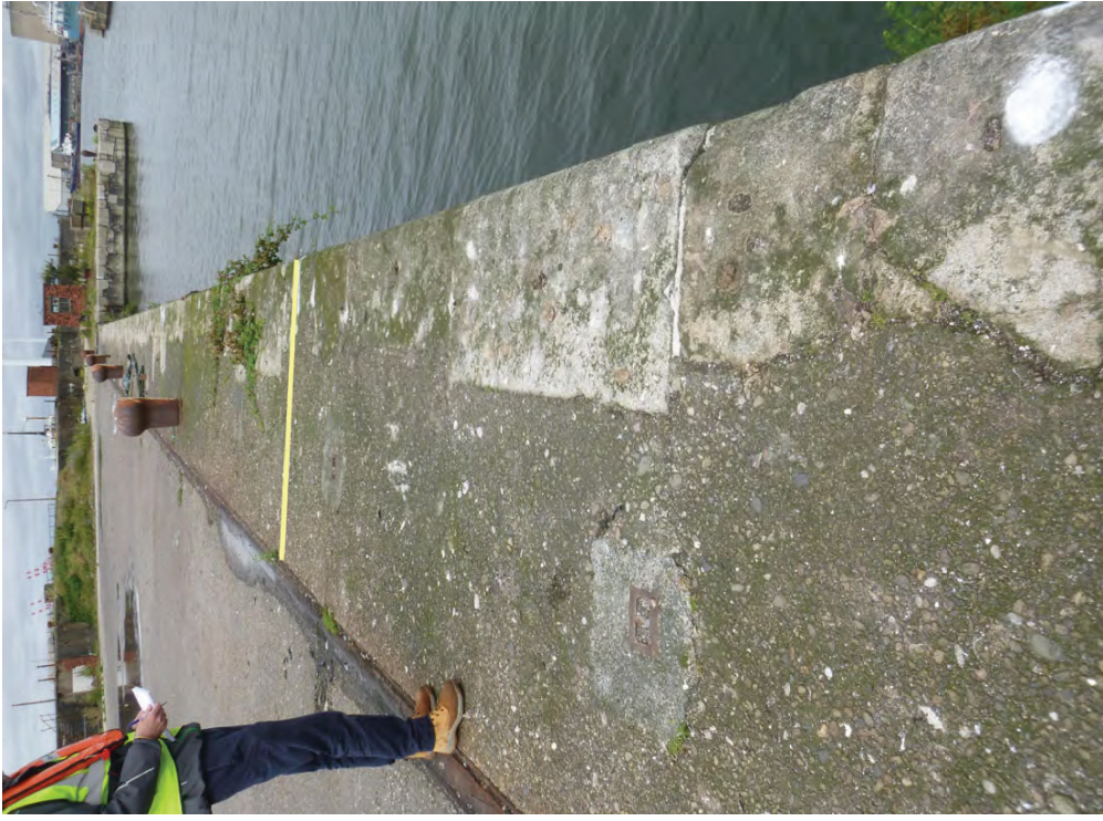
Figure A176a - Bramley Moore: Coping Chainage 855 to 860m
