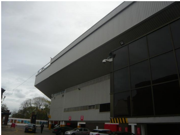
Photo C.1: Outside view of the Main Stand which is clad in corrugated metal.
