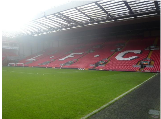
Photo C.6: The Kop is a single tier of seating which has multiple entry/exit points to the welfare areas behind.
