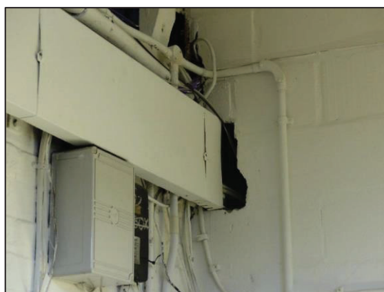
Photograph 17: Gaps in eastern wall of supporter access area in East Stand
