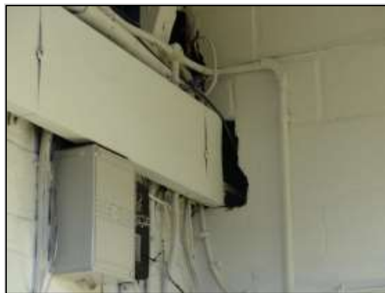
Photograph 17: Gaps in eastern wall of supporter access area in East Stand
