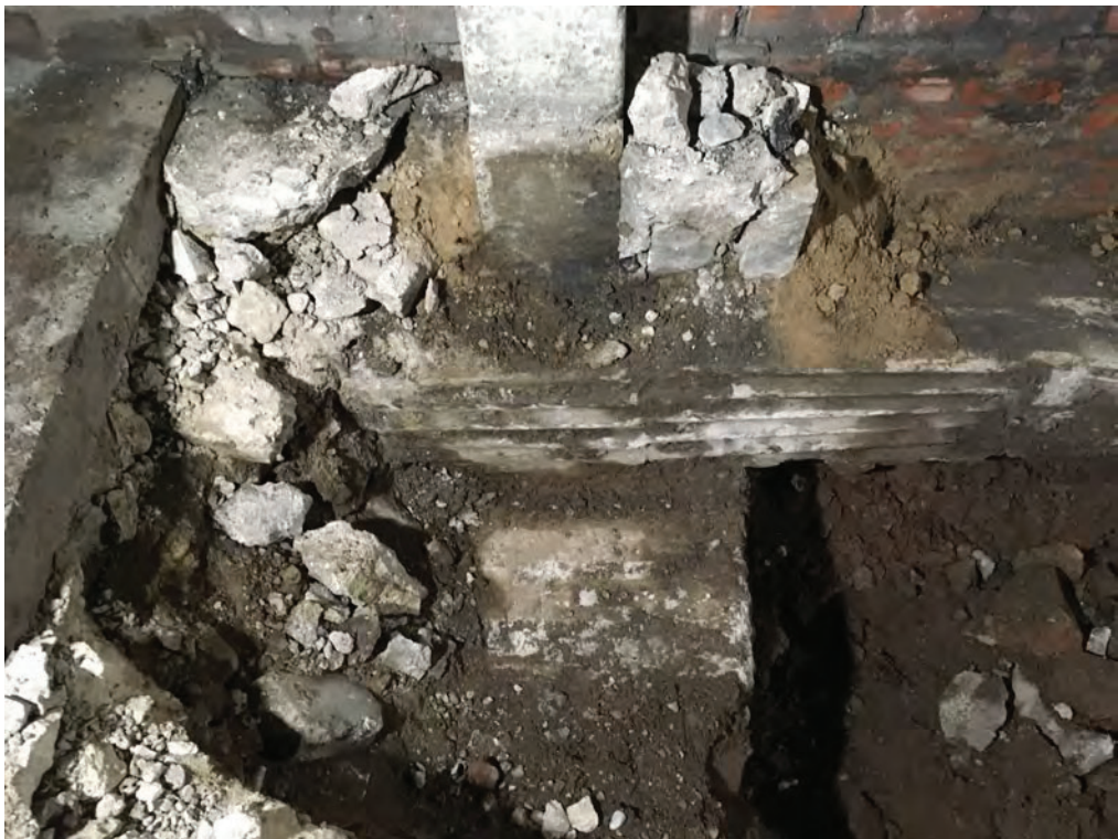
Western face, showing foundation and possible pile cap
