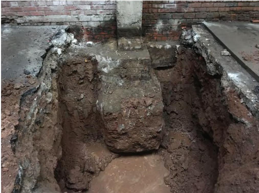
Excavated foundation and possible pile cap
