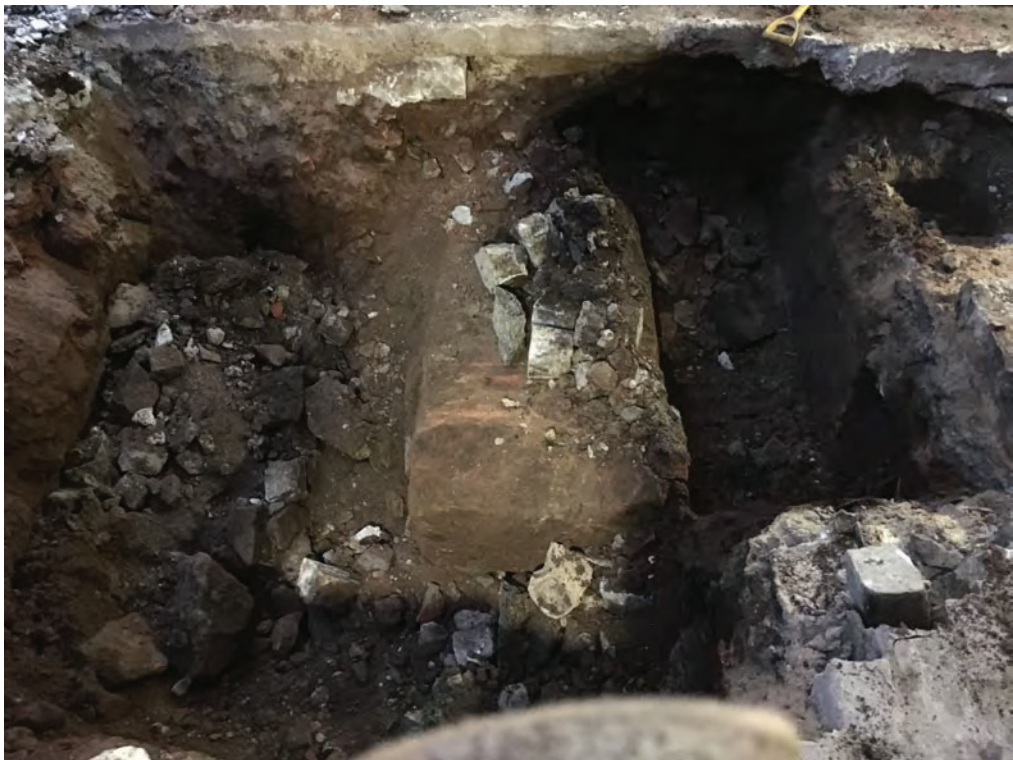
Eastern face (with sandstone block present, block excavated during trial pitting)
