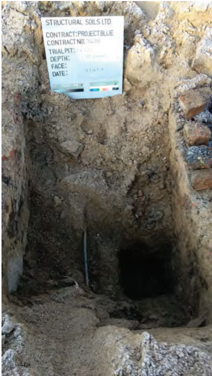
Pipework in southern part of excavation
