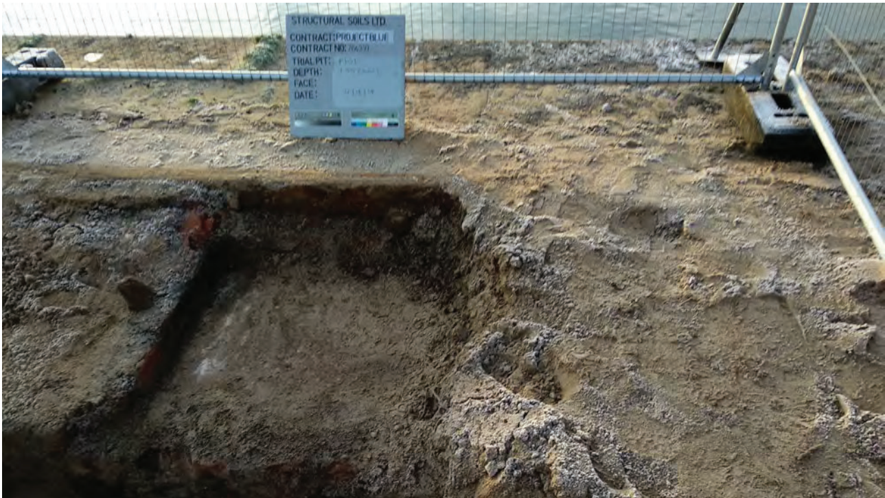
Southern part of excavation and rail
