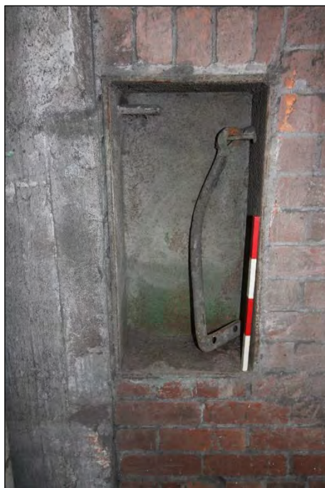
Plate 30: Steel box housing door retaining hook, with 0.4m scale
