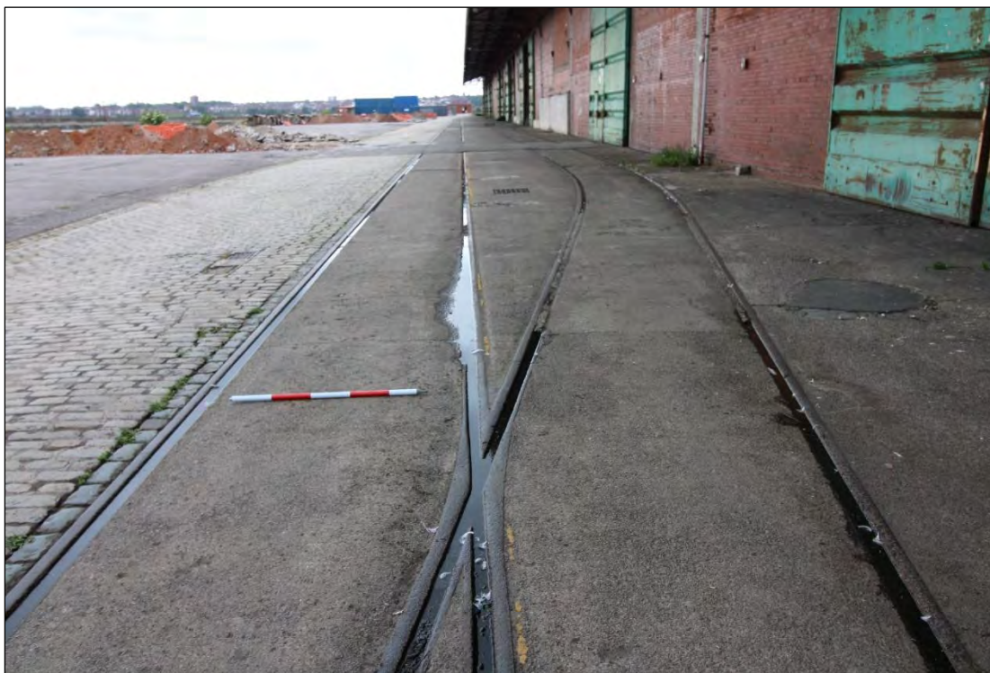
Plate 15: Grooved rails, passing the southern side of the Transit Shed, facing west with 1m scale
