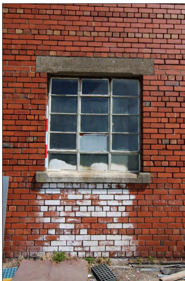
Plate 51: Typical Crittal-style window, on western elevation, with 1m scale
