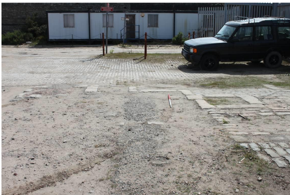
Plate 15: Infilled crane-base and areas of granite setts at the southern end of the eastern quay (Site 25)
