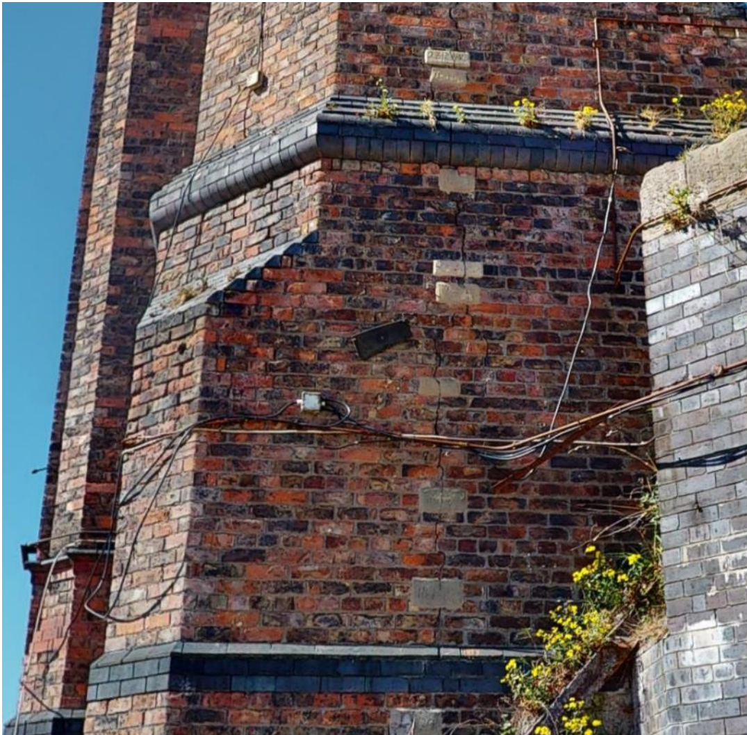
Figure 5: Coarse vertical cracking following the centreline of the facet panels of the chimney
