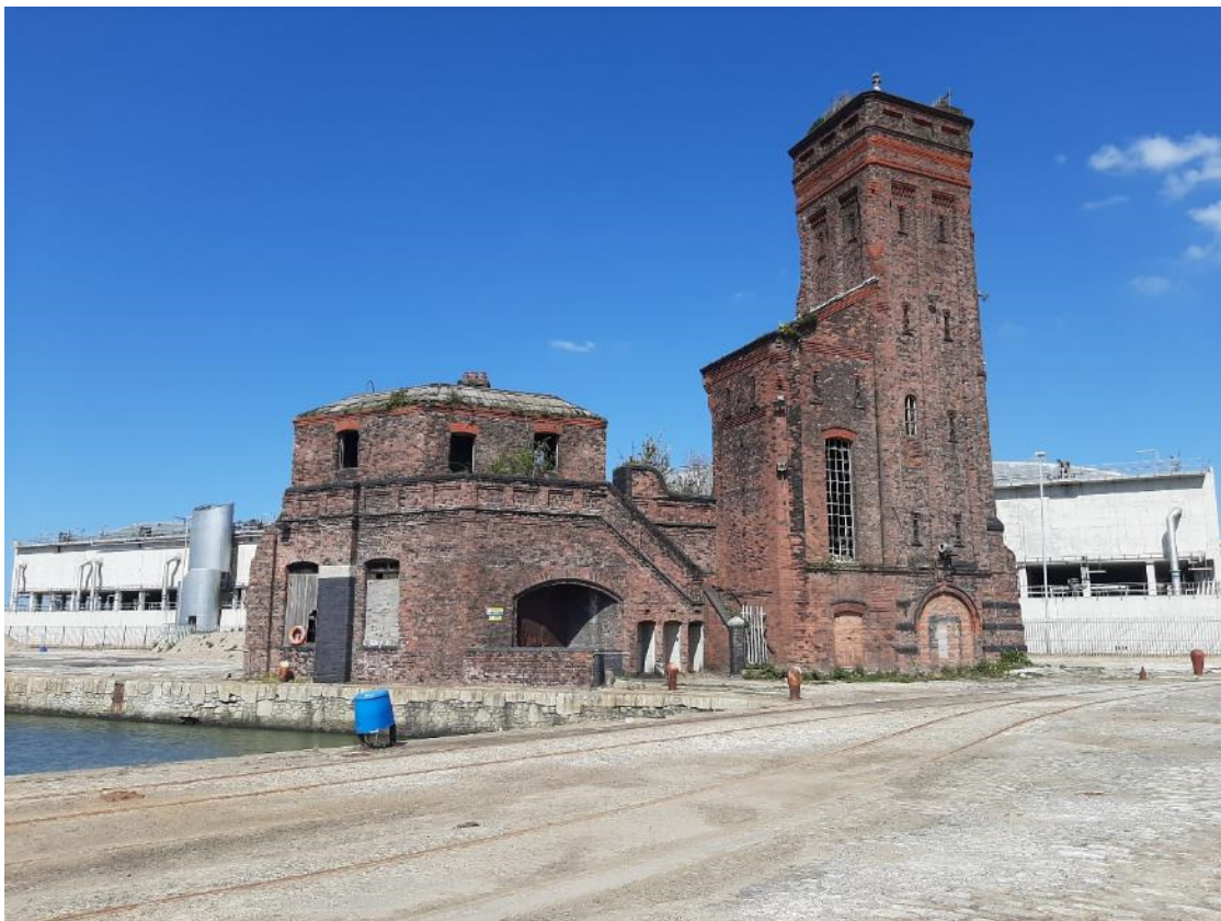
Figure 1: Hydraulic accumulator tower at Bramley-Moore Dock with integral boiler house (2020).
