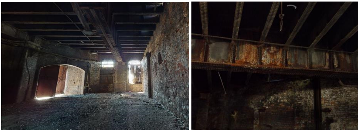
Figure 6: Internal images of the heavy-engineered roof deck over the Boiler House.
