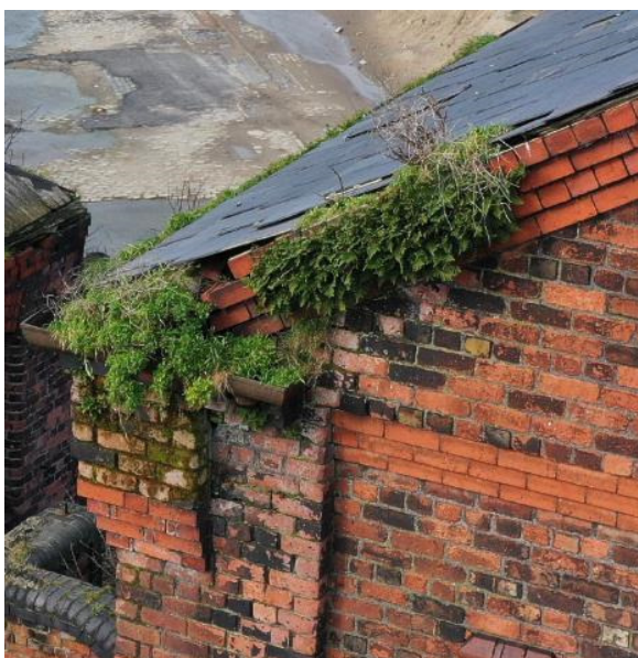
Figure 3: Fabric decay and vegetation particularly prevalent at structural elements which attract the wind
