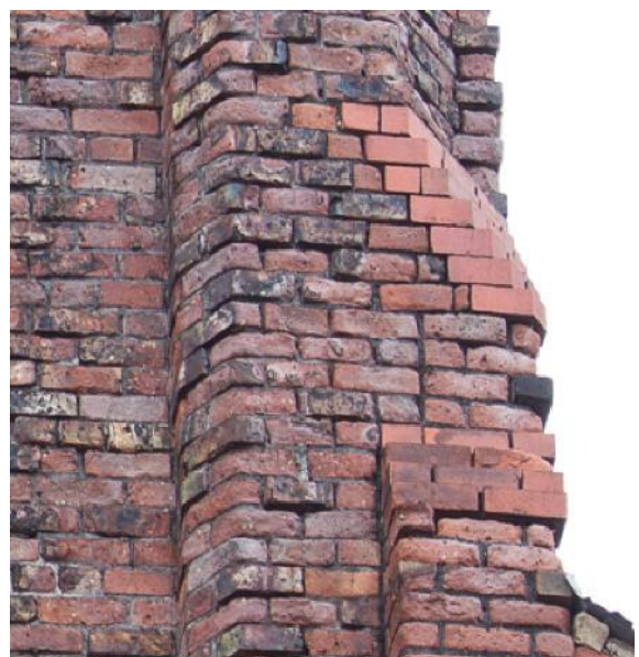
Figure 3: Fabric decay and vegetation particularly prevalent at structural elements which attract the wind
