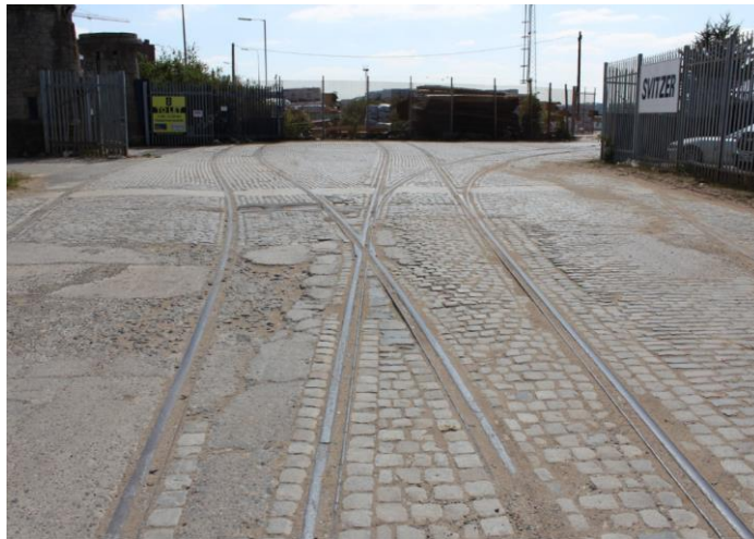
Figure 38: Bramley-Moore Dock: Granite setts and rail track
