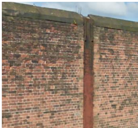
Figure 19: Cast iron railway stanchion
