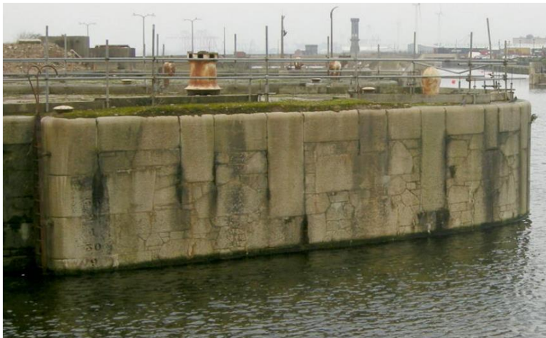
Figure 8: 'Cyclopean' Dock Retaining Wall
