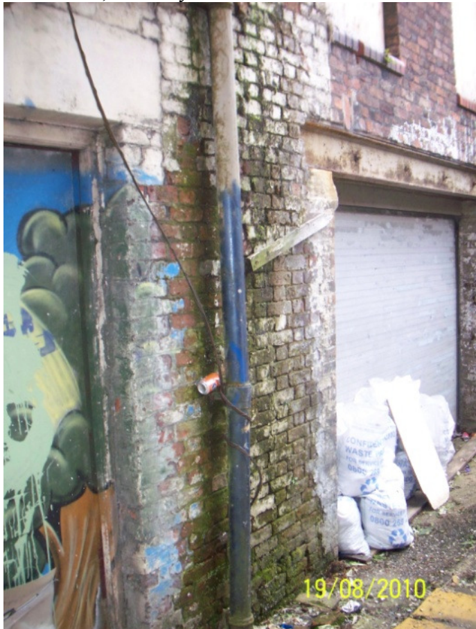
Photograph 6 – Defect 2, Loss of mortar in joints and vegetation growth
