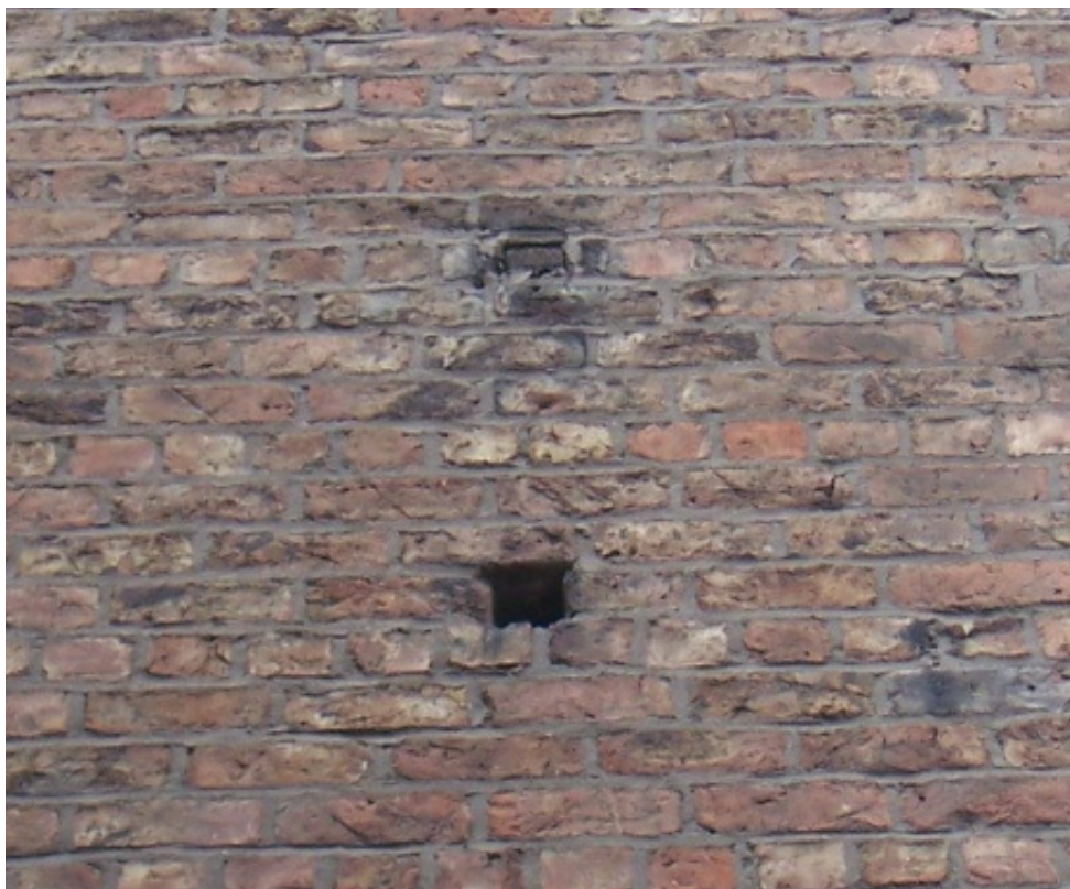
Photograph 3 – Defect 3, two holes in the masonry wall
