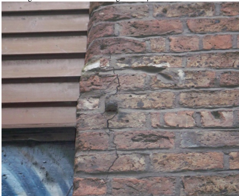
Photograph 1 – Defect 1, crack in the masonry external wall
