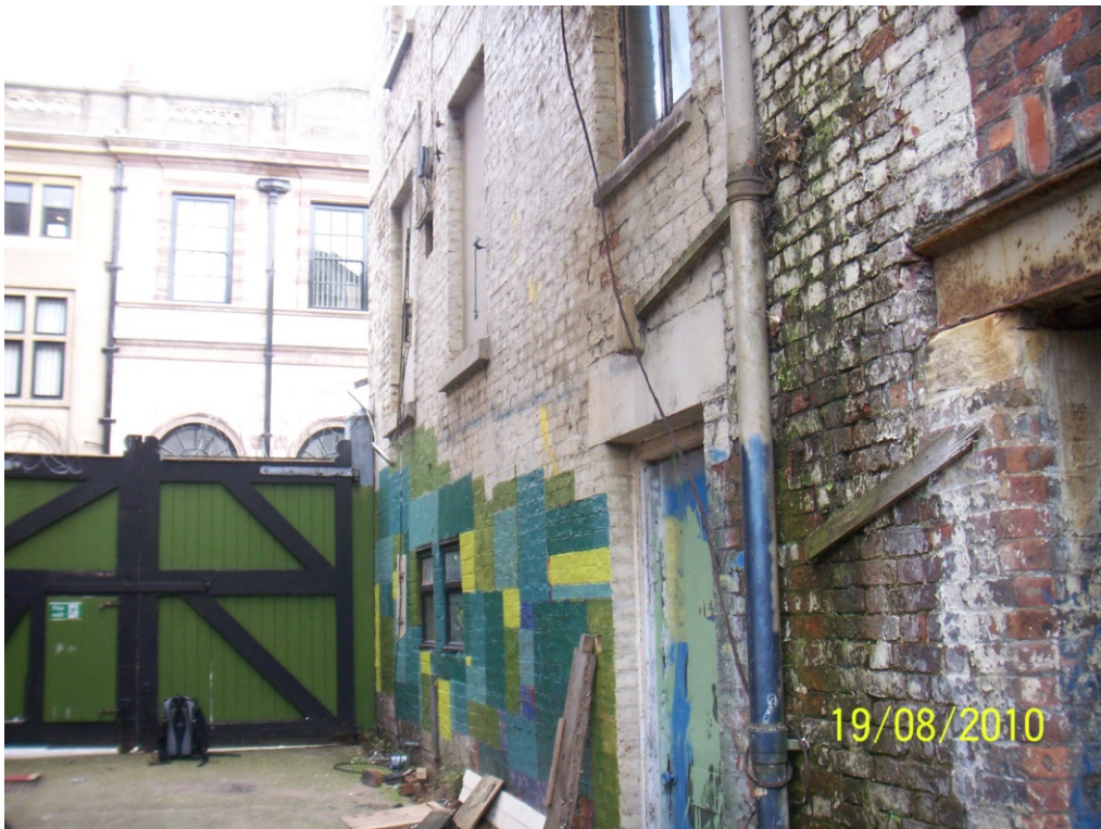
Photograph 5 – Defect 1, masonry cracks from window frame to concrete lintel
