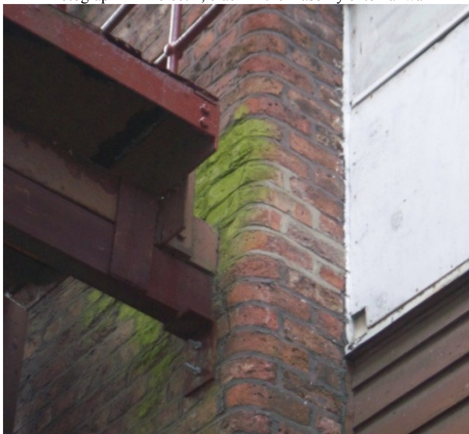
Photograph 2 – Defect 2, crack in the masonry external wall
