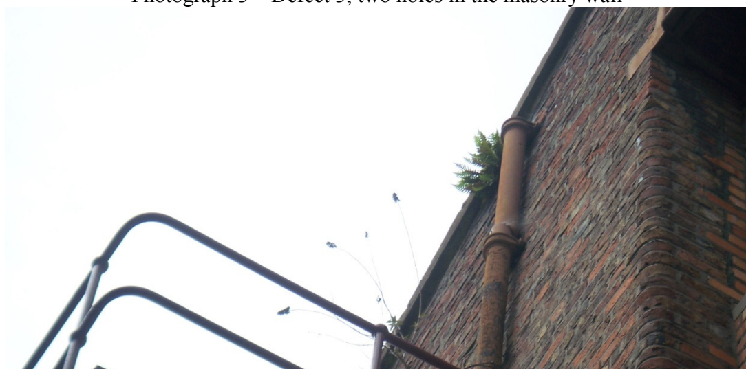
Photograph 4 – Defect 4, Vegetation Growth
