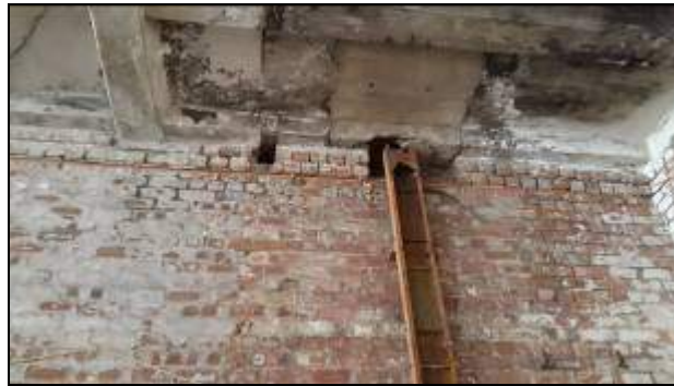
Photograph 17. Hole in brick wall on ground floor
