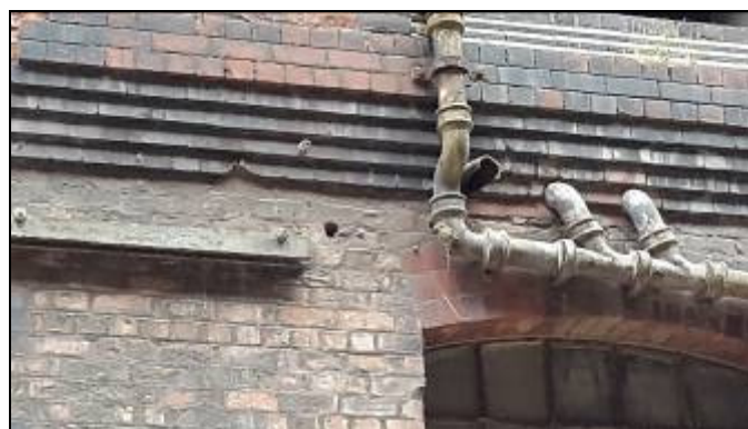
Photograph 14. Hole in brickwork where utility cable / pipe once entered wall cavity.
