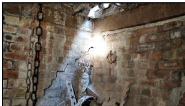
Photograph 20. Crack along brick wall within alcove in basement
