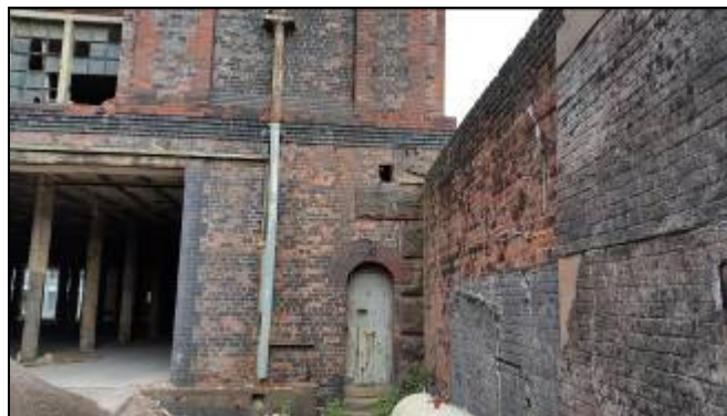
Photograph 13. Hole in brickwork where bricks have been removed.
