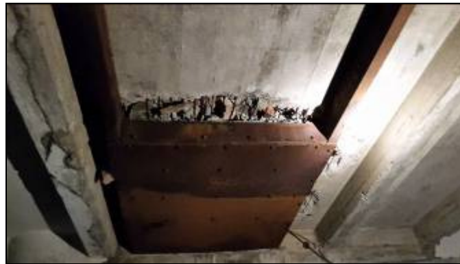
Photograph 22. Bricks / debris used to repair / fill hole in ceiling of basement.
