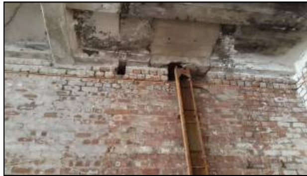
Photograph 17. Hole in brick wall on ground floor
