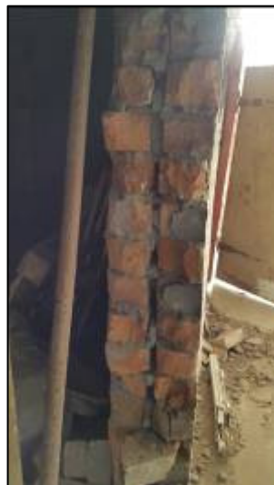
Photograph 18. Exposed wall cavity in brick wall on ground floor
