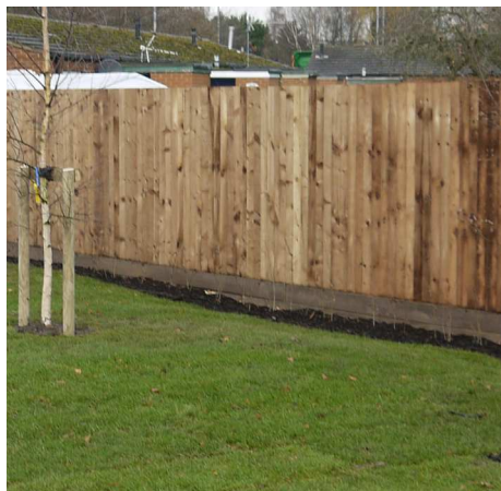
SAMPLE OF 1800mm HIGH CLOSE BOARDED FENCE
