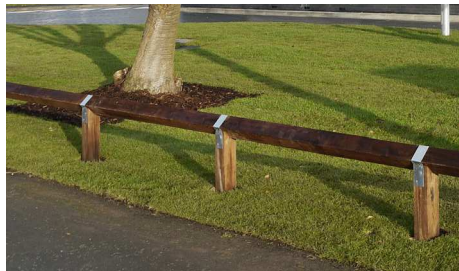
SAMPLE OF 450mm HIGH KNEE RAIL FENCE
