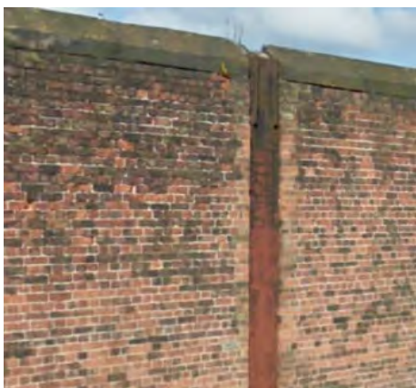
Figure 19: Cast iron railway stanchion
