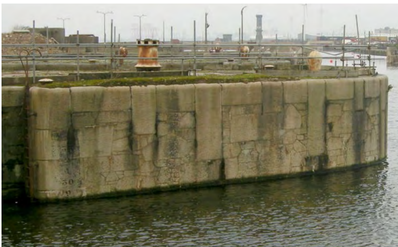
Figure 8: 'Cyclopean' Dock Retaining Wall
