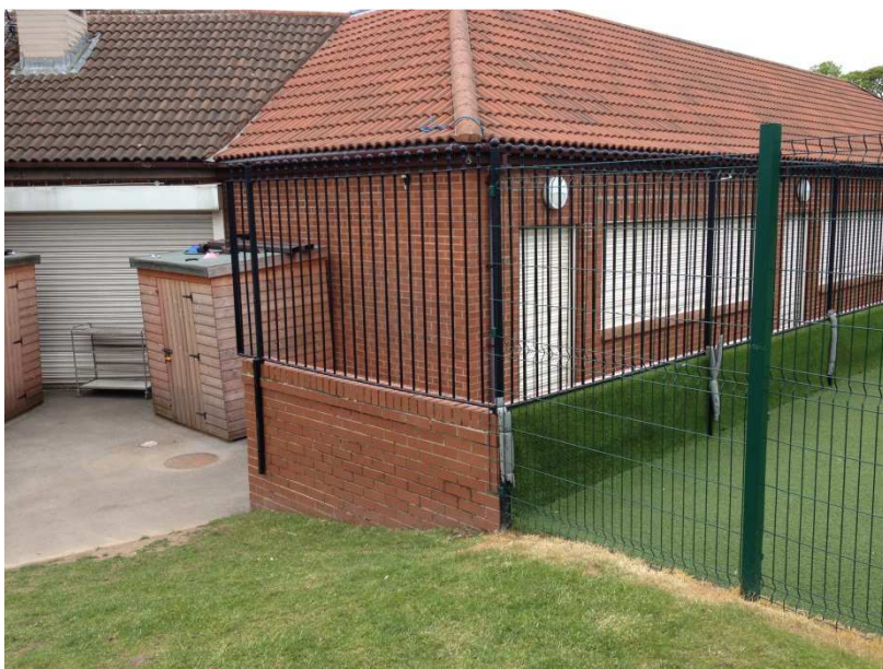
Fig.02-Existing retaining wall adjacent to kitchen area
