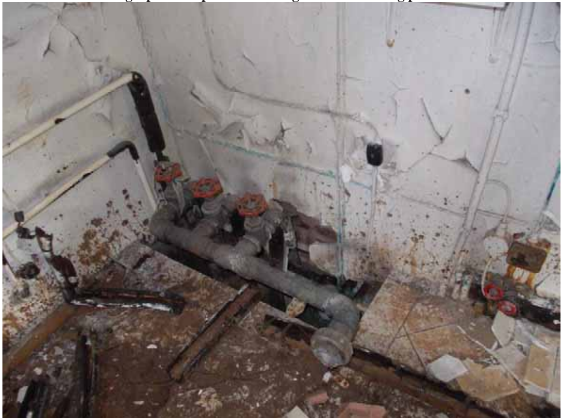
Photograph 20: Pipework relating to the swimming pool boiler
