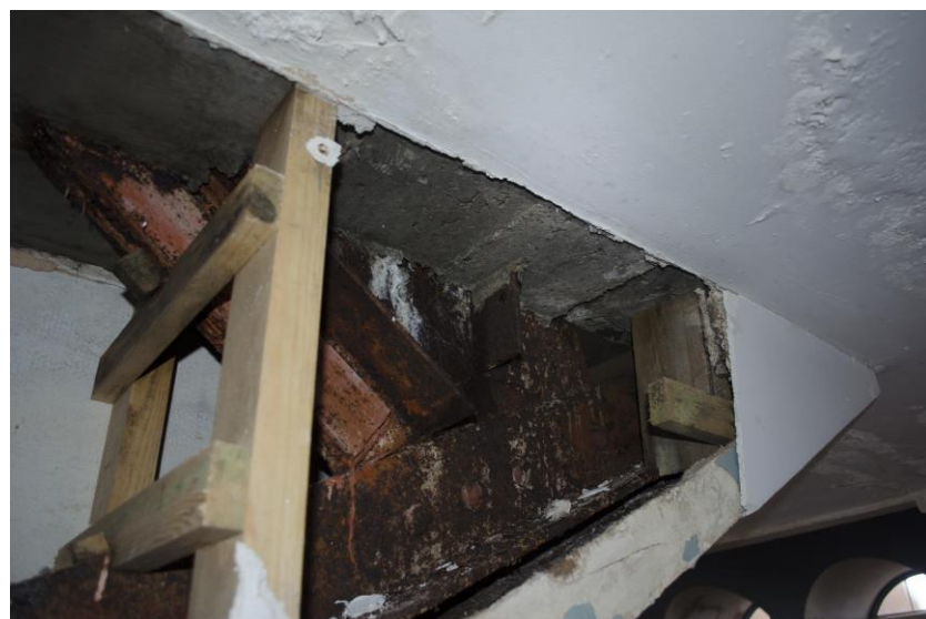
Figure 15 Exposed internal truss end showing retrofitted steel
