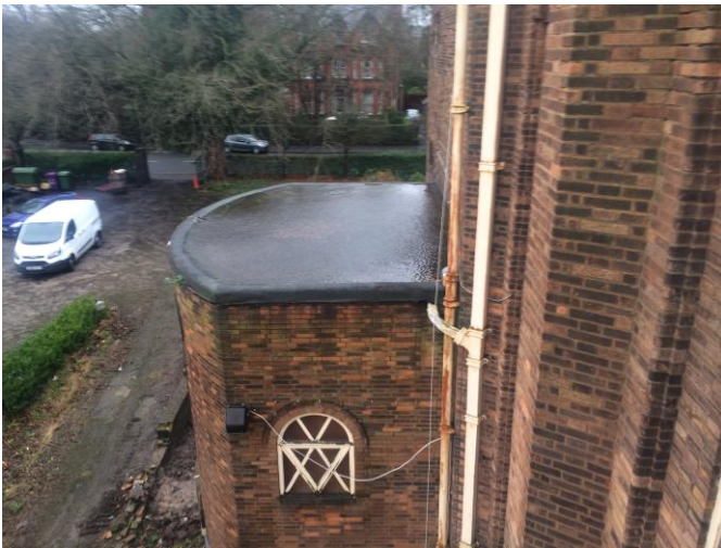
Figure 10 Ponding of water on flat roofs.
