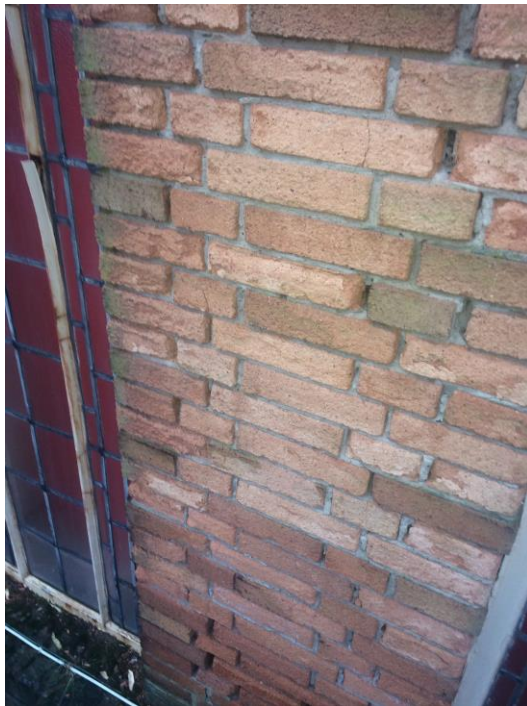
Figure 6 Eroded and frost damaged masonry
