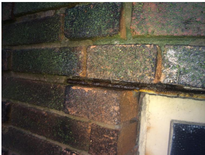
Figure 3 Corroding window lintel
