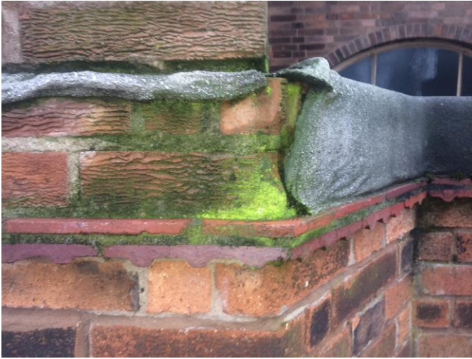
Figure 9 Failed or poor detailing of roof coverings leading to water ingress.
