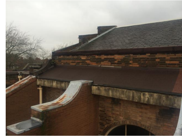
Figure 11 Flashings in lead and flash band. Note ridge formed in folded plastic or metal sheet.
