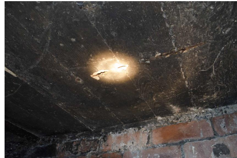
Figure 11 Reinforcement exposed
