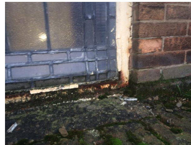
Figure 8 Corrosion to window frame and bulging of leaded window glazing.
