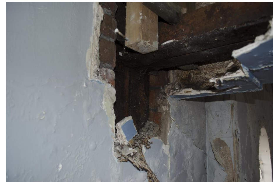
Figure 14 Exposed internal truss end
