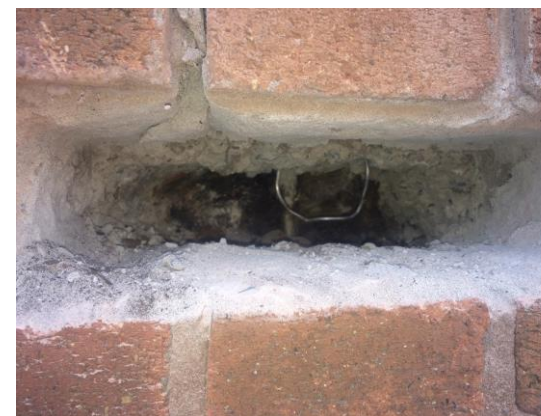
Figure 5 Exposed Steel Channel Columns to external masonry columns
