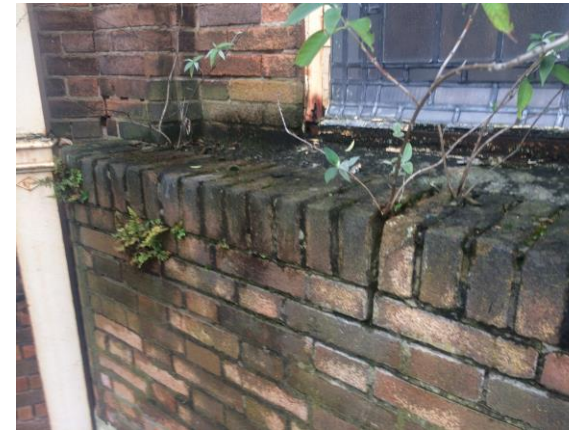
Figure 7 Masonry window box feature note damage and concrete infill to top.
