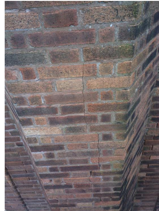
Figure 4 Cracking to external masonry columns
