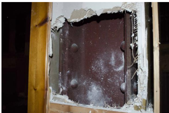
Figure 12 Exposed Internal Column
