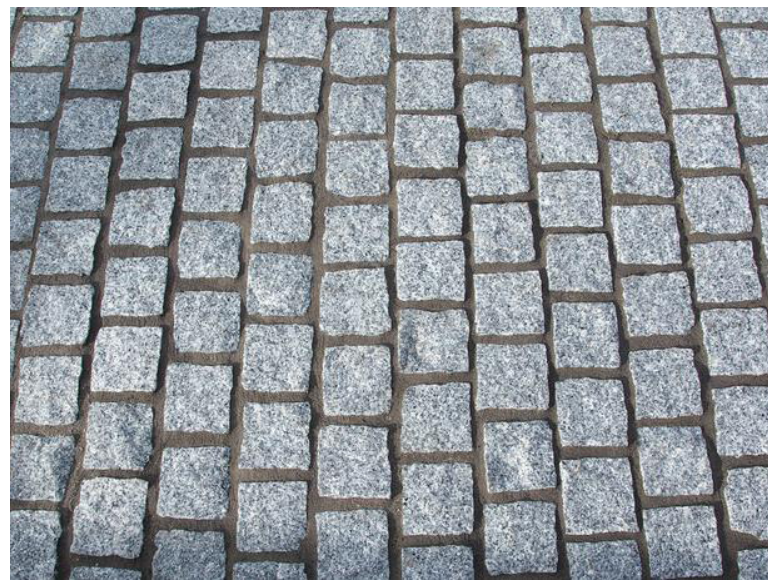
Cropped surface units used to deter skate boarders and as an edging detail
