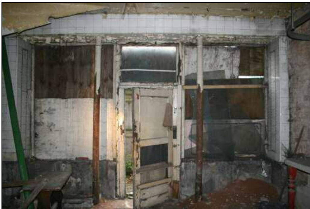
Shop front from interior showing cast iron columns and white tiled reveals
