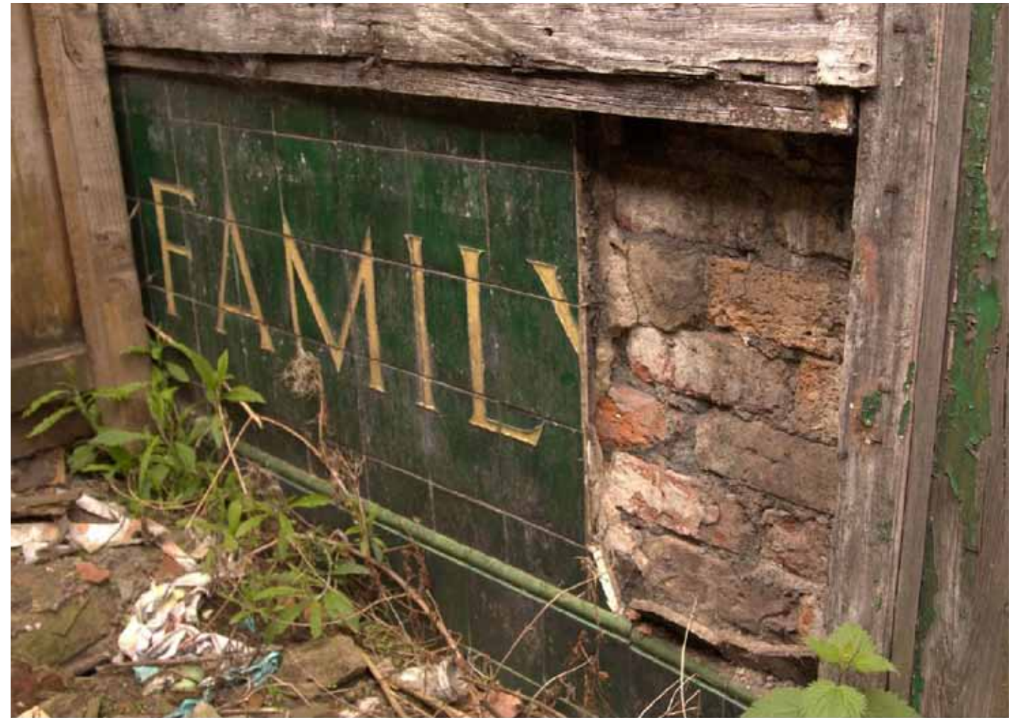
Photograph 7 View showing the condition of the brickwork behind the tile finish.
