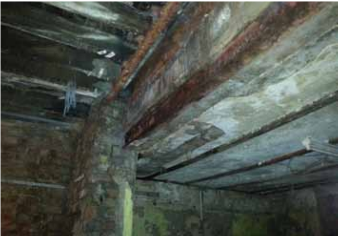
Ground Floor - Damaged structural beam
