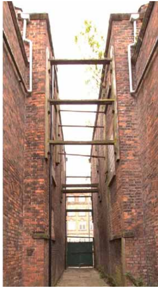
Photograph 1 View looking along the alley between the Bookshop and No 39. Note the flying shores are timber and are relatively simple in form. The walls on both sides appear to be out of plumb.
