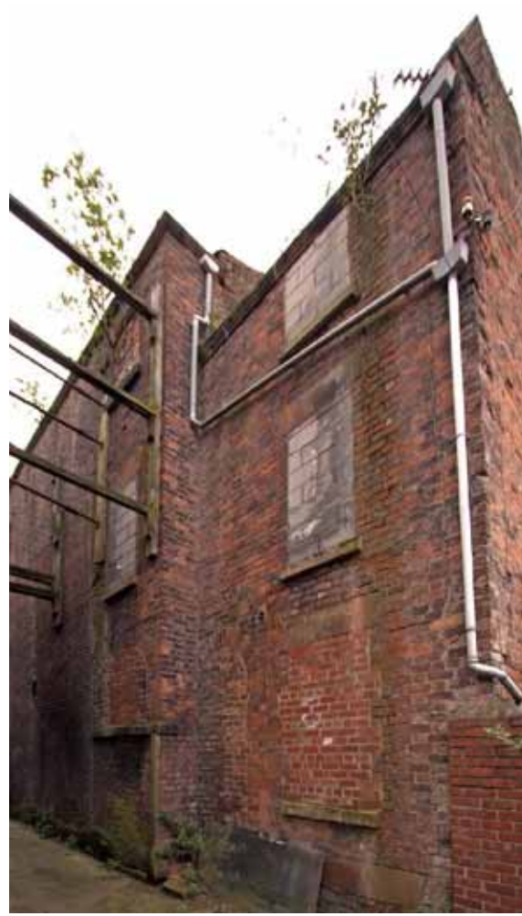
Photograph 2 View looking onto the side wall of the Bookshop showing the original entrance doorway (now infilled), the flying shores, areas where brickwork appear to have been modified, vegetation at roof level and replacement guttering.
