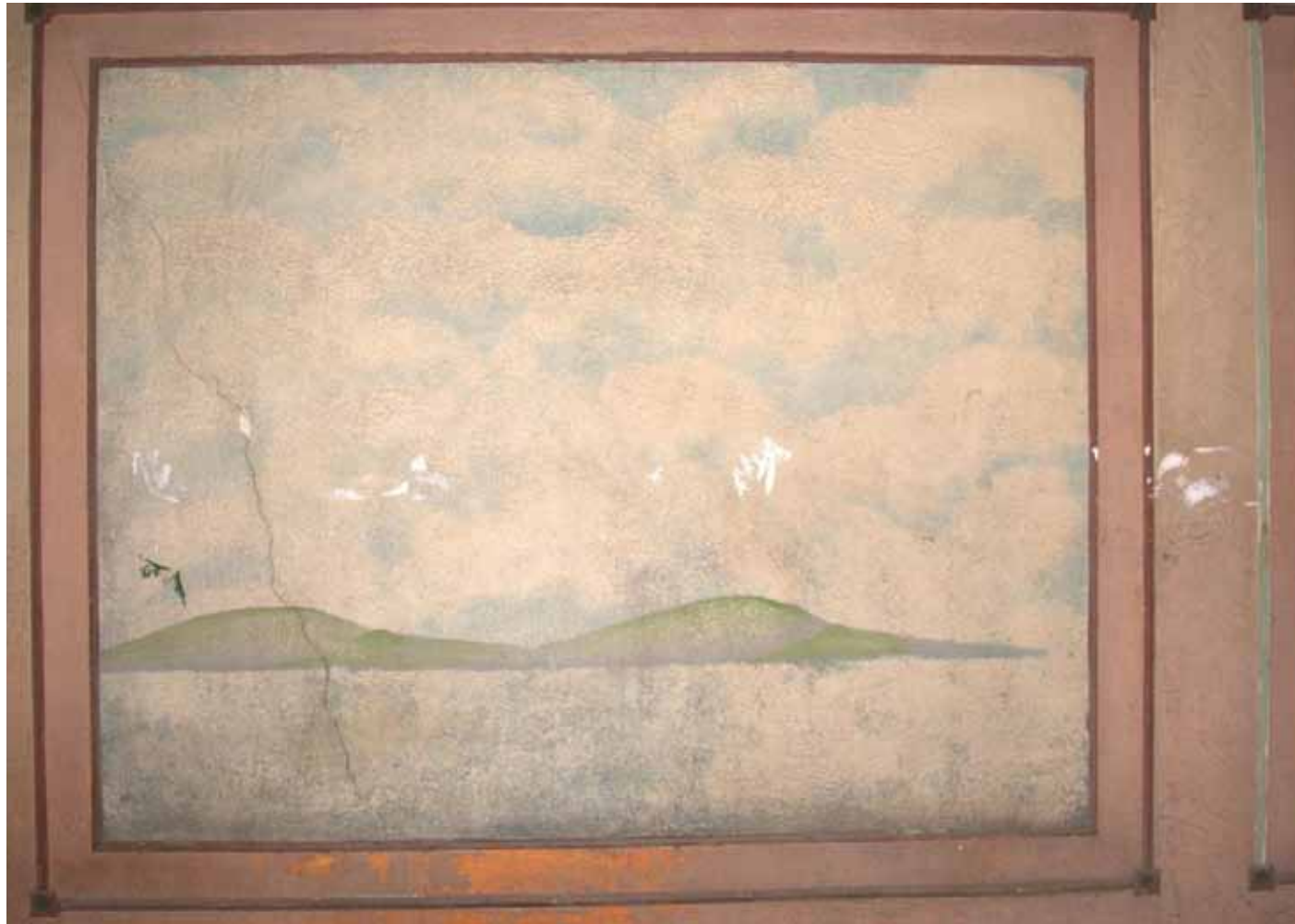
Photograph 6 View at 1st floor showing cracking across the painting which is a result of outward movement of the gable front elevation with respect to the flank wall.
