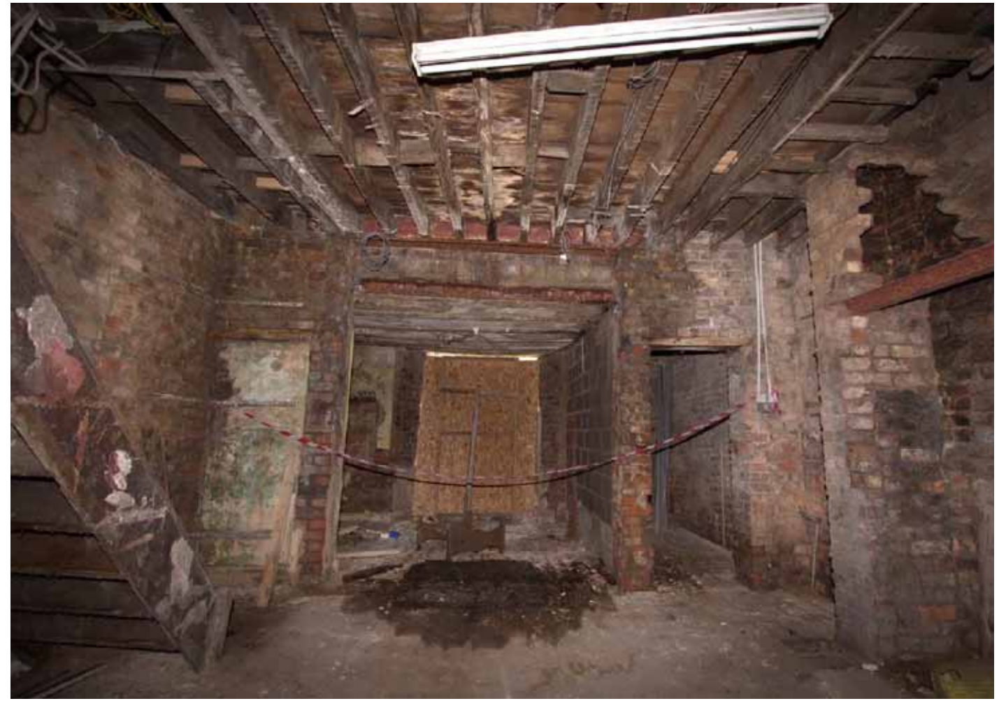
Photograph 3 View on the inside of the upper level of Galkoffs showing saturated floors, corroded steel beams, concrete roof slab to outrigger extension; replacement staircase, modified chimney breast and water staining on the first floor.
