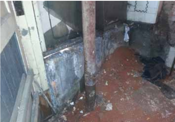
Ground Floor - Damaged structural beam
