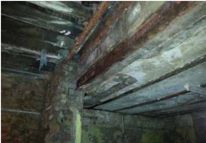
Ground Floor - Damaged structural beam
