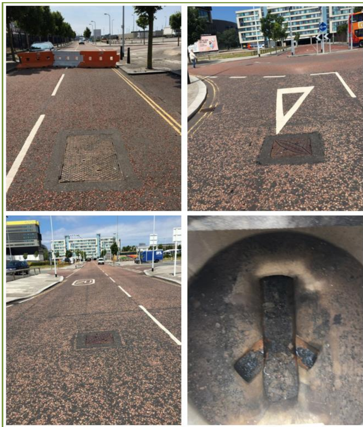
Top Left: Foul manhole SW19 looking west along Half Tide Wharf Top Right: Surface Water Manhole SW10 looking north to Queens Wharf Roundabout Bottom Left: Manhole SW12 looking North Bottom Right: Inside of Manhole SW10 showing connection spurs
