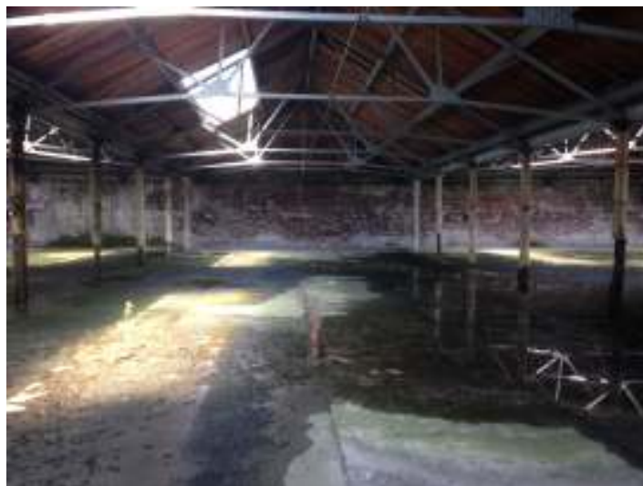
Photo 6: Angle Iron Roof Trusses
