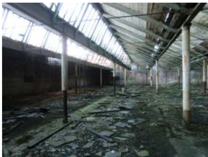
Photo 10: North Light Roof Trusses
