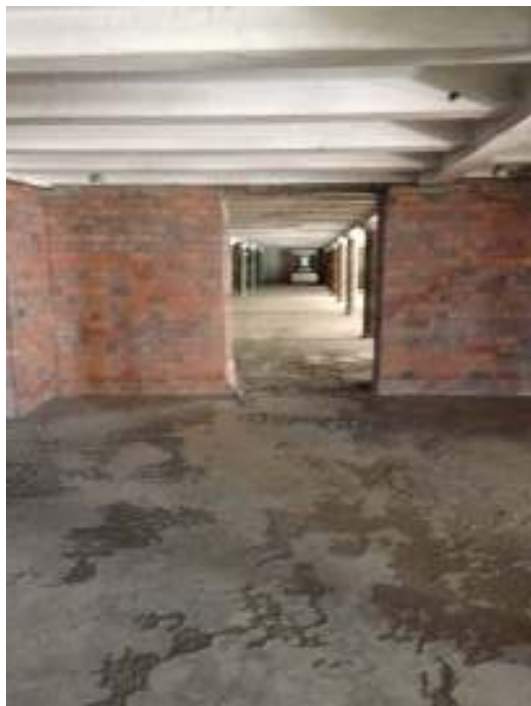
Photo 9: Masonry cross walls
