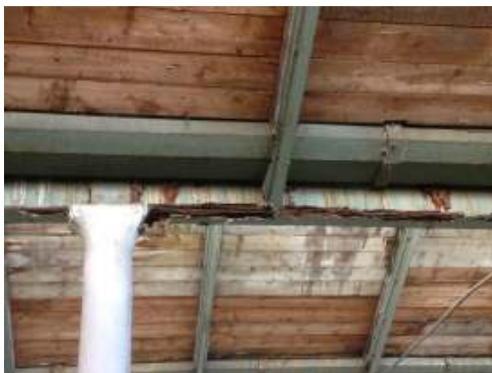
Photo 8: Deterioration around roof column and beams
