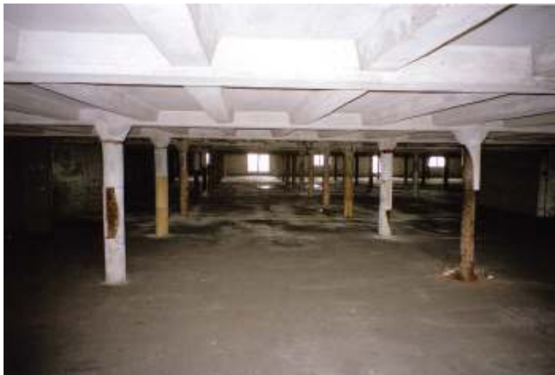
Photo 3: Typical floor structure showing down stand filler joists and
