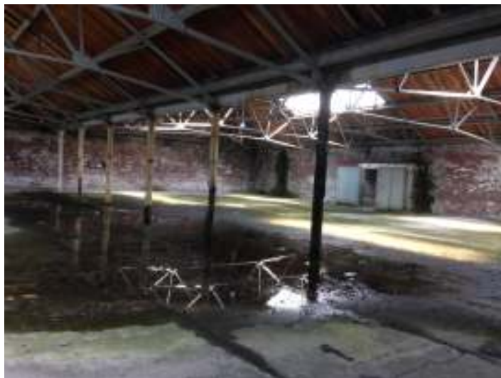
Photo 7: Water on slab on existing level 12
